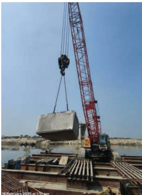
Fig.6: A diamond-wire-cut concrete prism (1.0 m × 1.0 m × 3.0 m, ~7.5 tonnes) being lifted vertically from the well cap by the barge-mounted crane. The clean planar faces produced by wire saw cutting are clearly visible.
