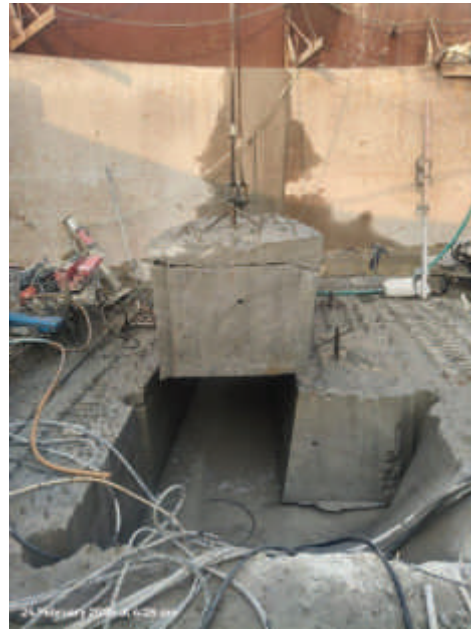
Fig.7: Close-up view inside the well cap during extraction (24 February 2026). The precision planar faces of the diamond wire saw cuts are evident on both the extracted block and adjacent cut surfaces. Diamond wire saw machine and hydraulic hoses are visible in the foreground.
