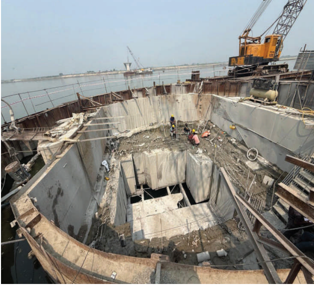
Fig.8: Intermediate stage of well cap removal showing several prisms already extracted, revealing the sacrificial steel truss at the base. Remaining prisms, some mid-cut, are still in place. The barge crane is visible at upper right, and two pylon shafts of adjacent piers are visible across the river.
