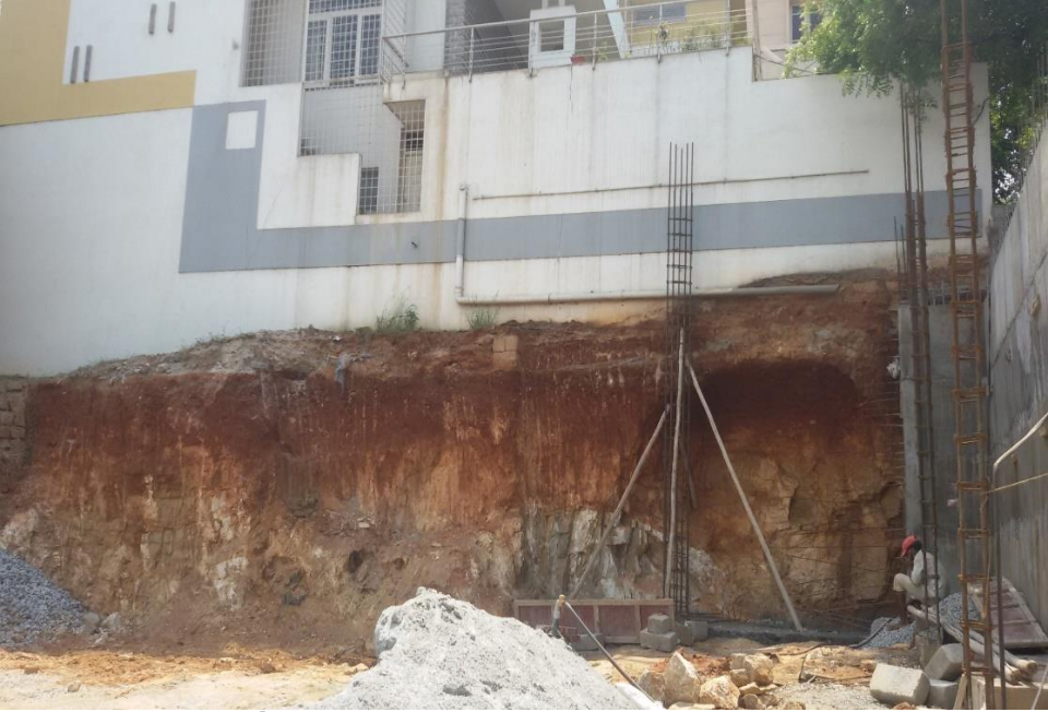
Excavation under the compound wall
