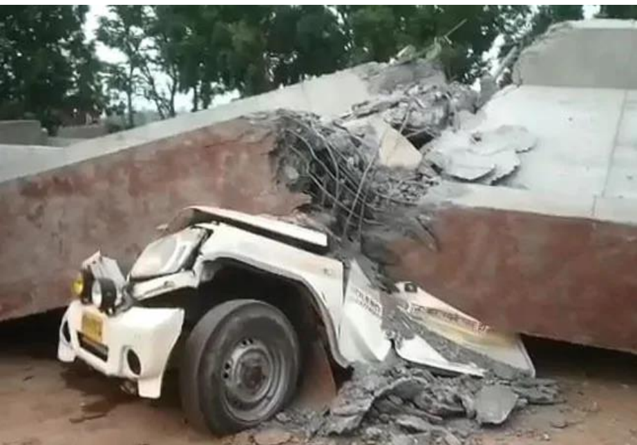
Flyover, Under Construction, Collapses in Gurgaon, UP
