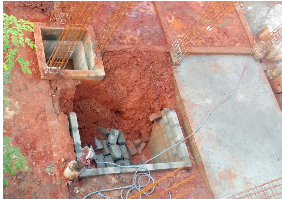
Collapse of sump tank wall
