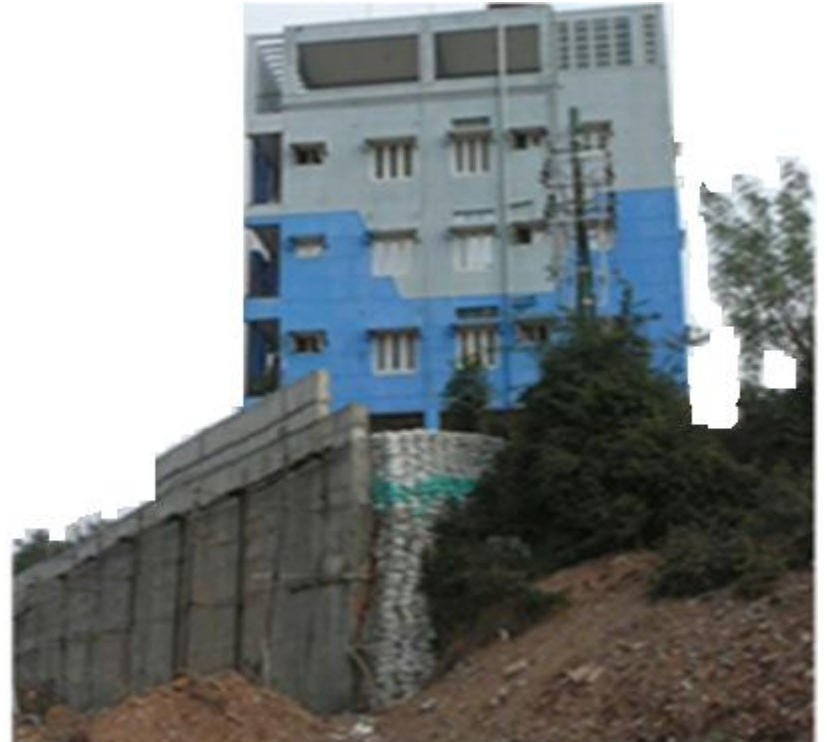
b) View of an existing structure
