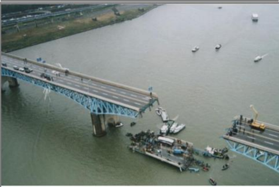
Seongsu Bridge after collapse (Seoul, South Korea, 1994) Han river: 6 cars fell, 32 killed, 17 injured
