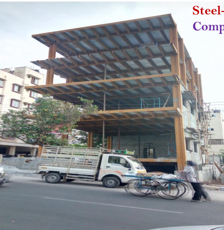
Metal decking in a Floor construction
