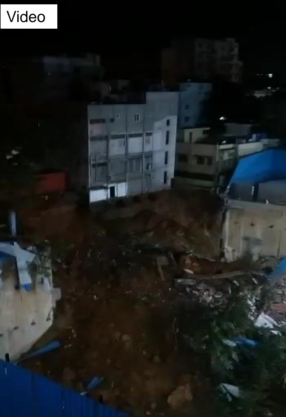
Three storey building behind the under construction site collapsed on July 28, 2020 , 50 feet deep basement in the adjacent site
