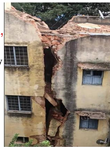
Collapse of Staircase passage of a three storey staff quarters building of Bengaluru Milk Union near diary circle on 28-9-2021
