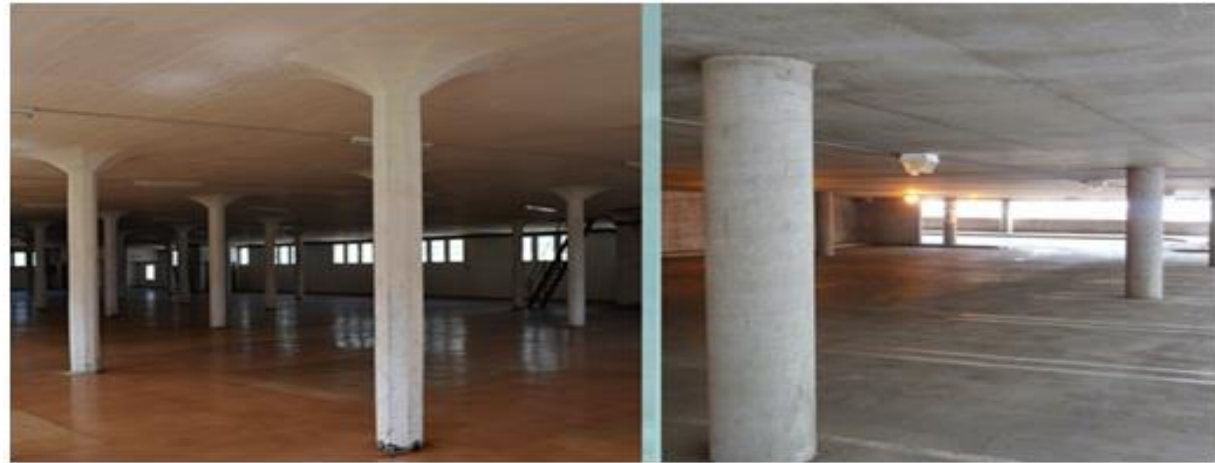
Flat Slab Vs Flat plate Slab
