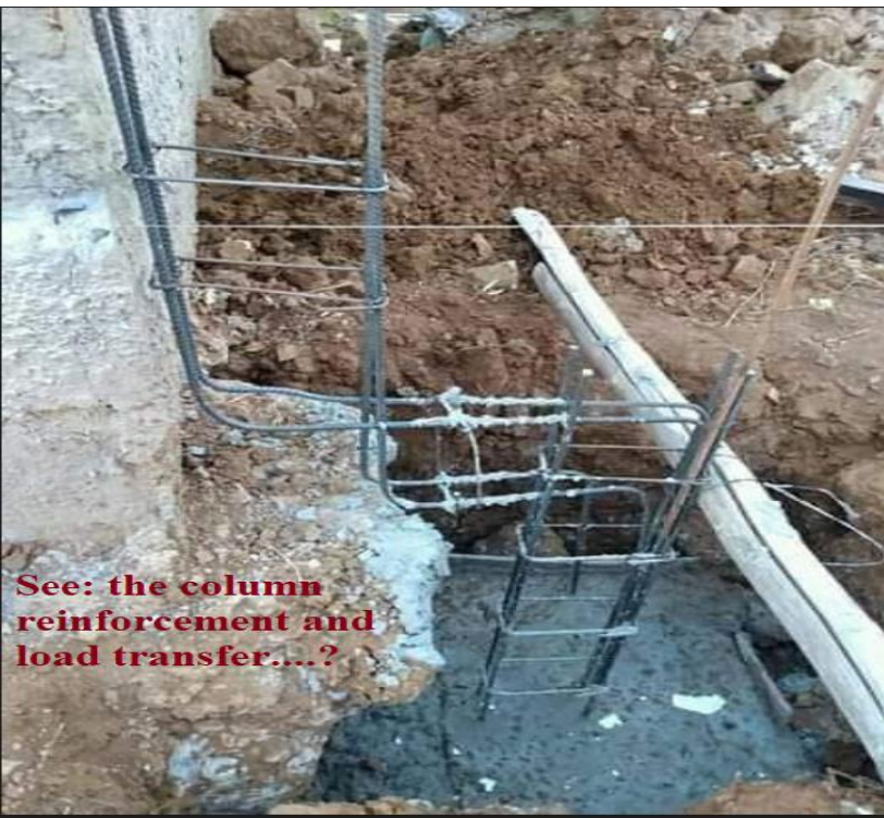
Excavation under the compound wall
