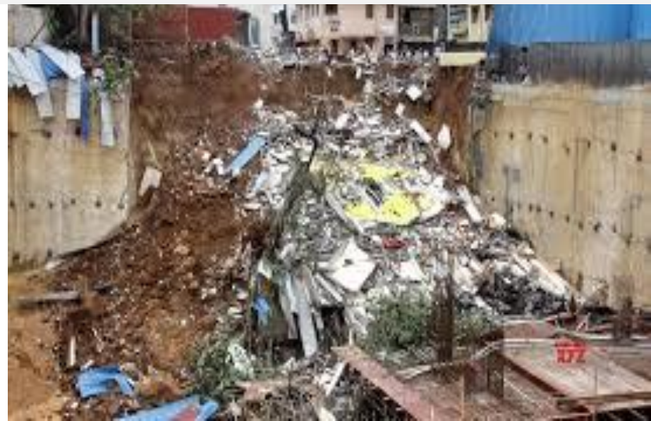
Three storey building behind the under construction site collapsed on July 28, 2020 , 50 feet deep basement in the adjacent site
