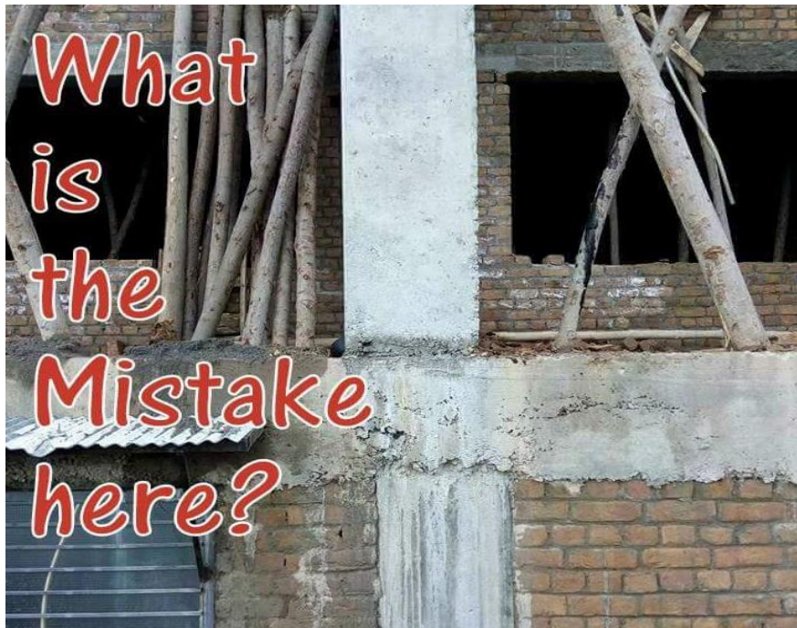
Column misaligned... poor substitute
