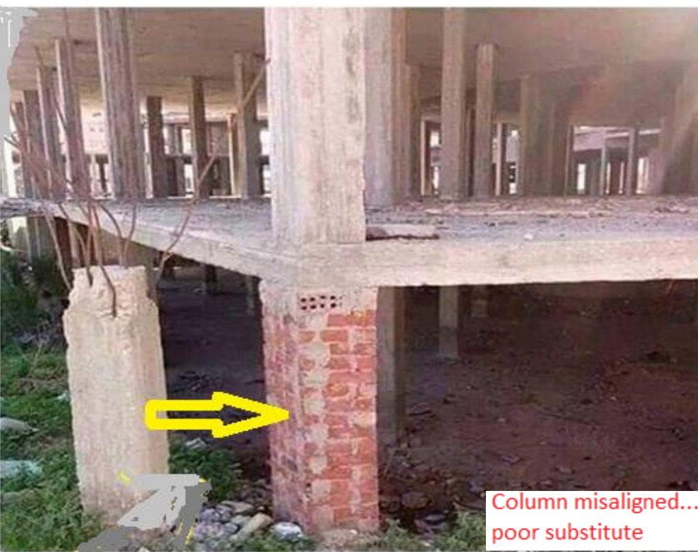
misalignment of beam and bad concreting for column
