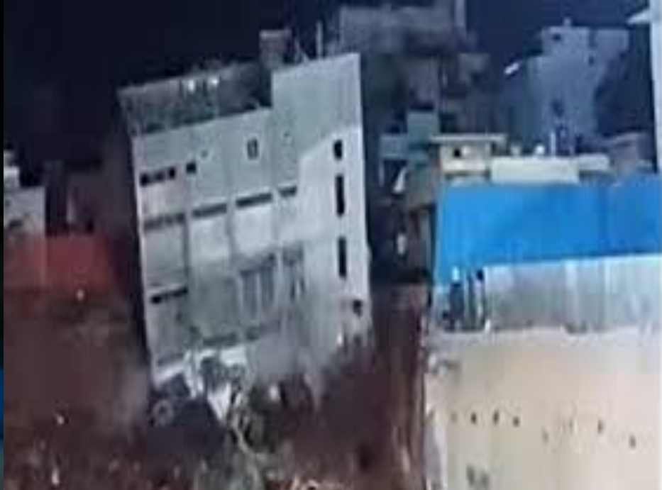
Three storey building behind the under construction site collapsed on July 28, 2020 , 50 feet deep basement in the adjacent site
