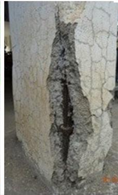
Cracks in columns due to corrosion expansion
