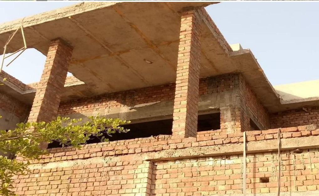
Column misaligned... poor substitute
