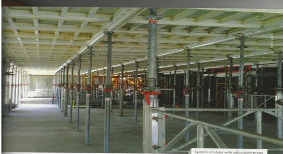
System of slabs with adjustable props
