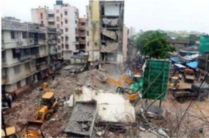
Waste is created from non engineered poor quality construction
