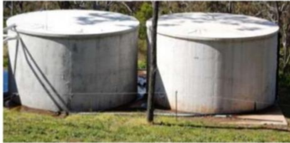
Figure : INSITU Water Tanks With Blended Concrete (Left) And Geopolymer Concrete (Right)
