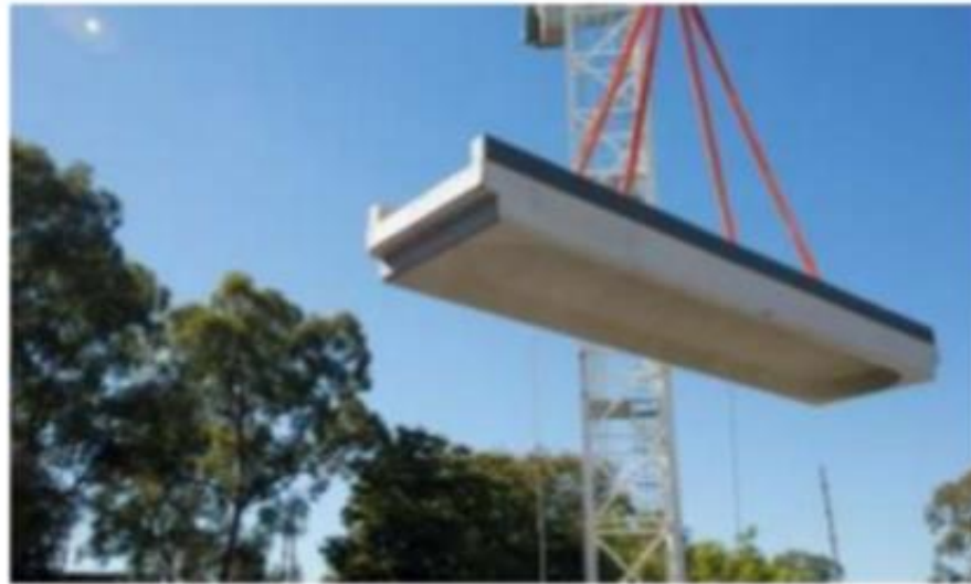
Figure : GEOPOLYMER CONCRETE BEAM CRANED TO POSITION
