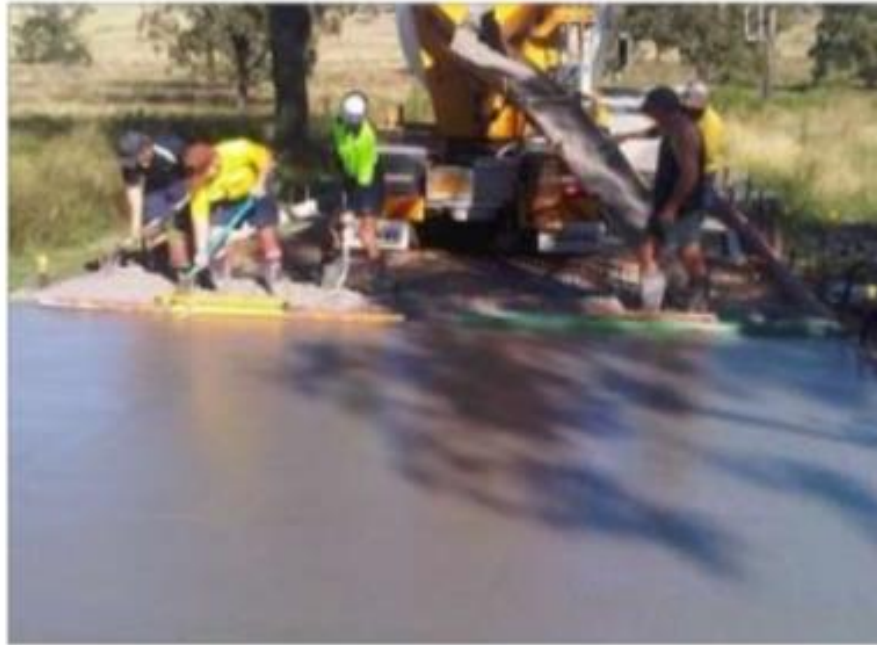
Figure : Placing of Pavement Using Geopolymer Concrete
