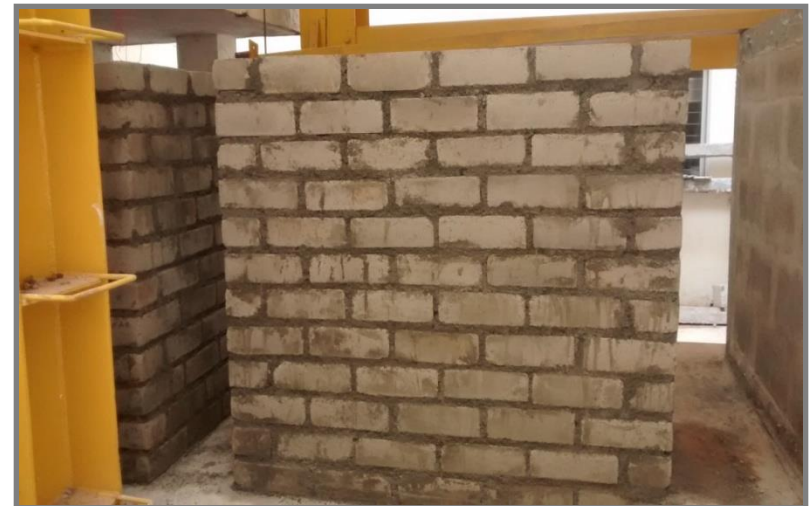
Stretcher Bonded Geopolymer Brick Wallete kept for Curing
