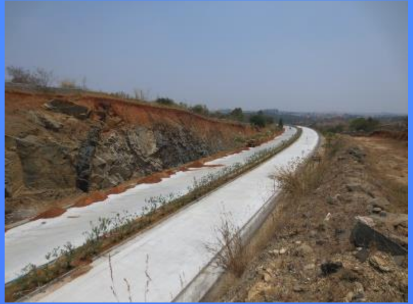
Over View of Finished Rigid Pavement
