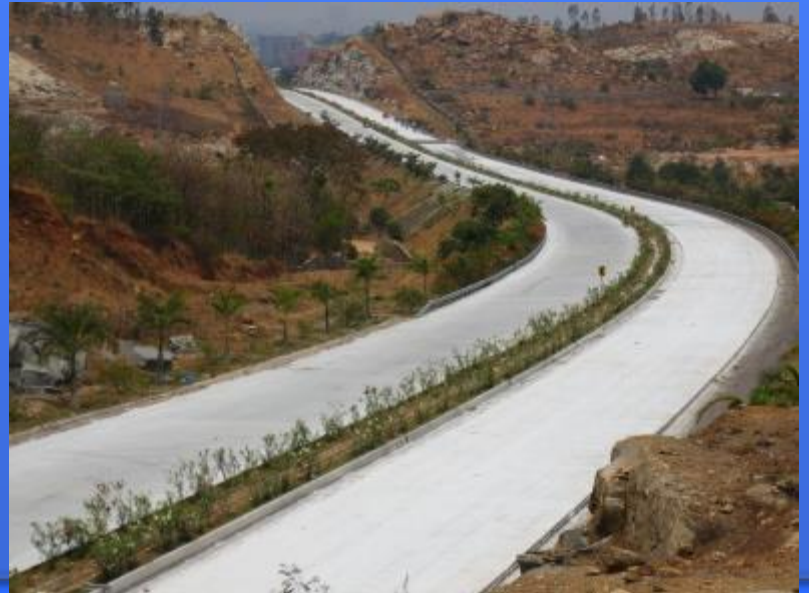
Over View of Finished Rigid Pavement
