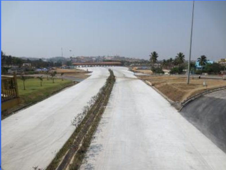
Over View of Finished Rigid Pavement
