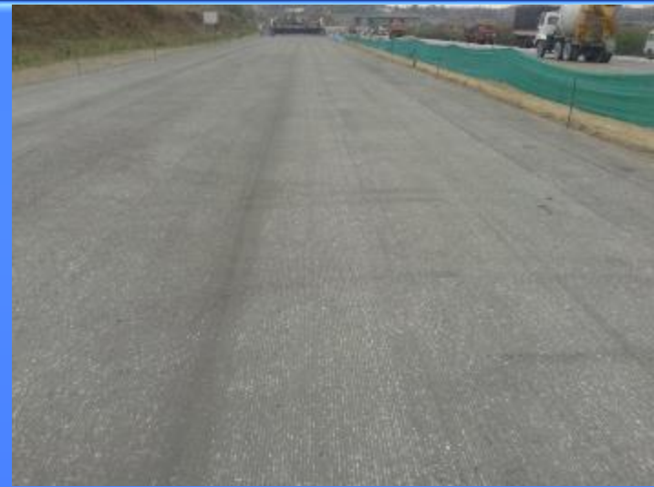
Milled Bituminous surface
