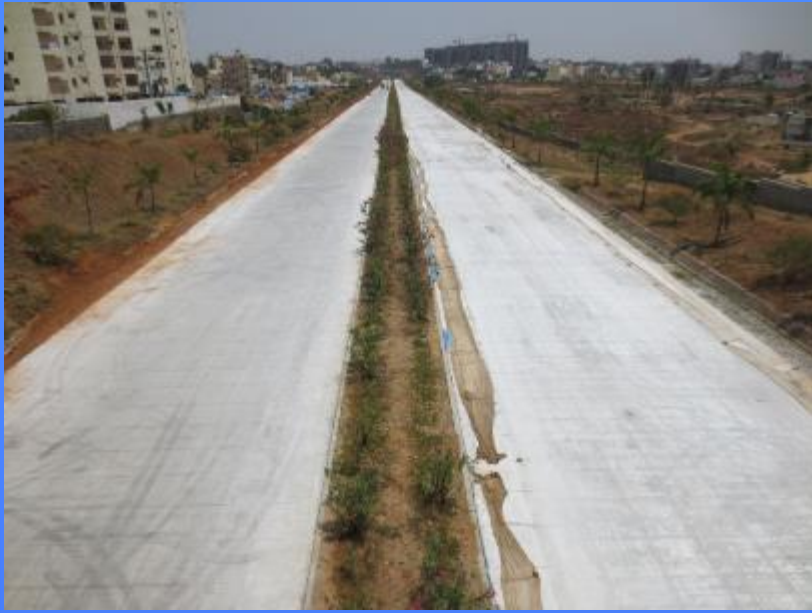
Over View of Finished Rigid Pavement
