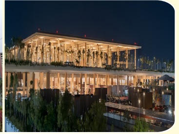
2024 - Construction of Terminal 2, KIAL
