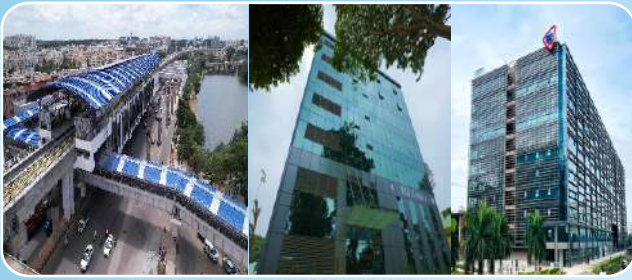
2023 Construction of Elevated Viaduct & Station for Bangalore Metro,
