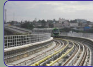
2014 - R3 Phase I B'lore Metro Project
