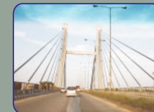
2003 - Cable-stayed bridge at K. R. Puram, Bangalore
