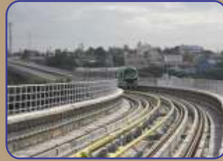
2014 - R3 Phase I B'lore Metro Project
