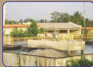
2004 - Waste Water Treatment Plant, Mylasandra, Bangalore
