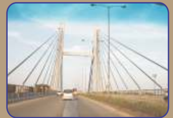
2003 - Cable-stayed bridge at K. R. Puram, Bangalore
