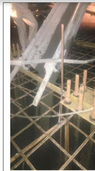
Footing Concreting
