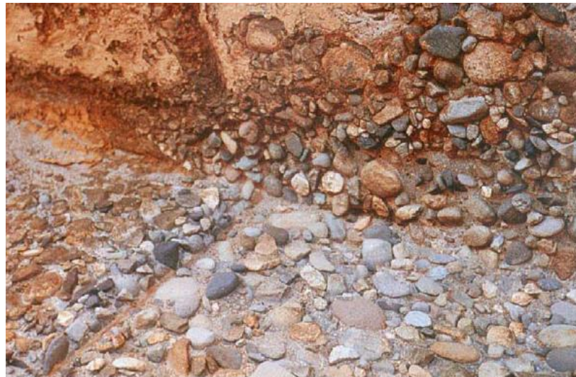
Figure A.4.2.1 Disintegration by chemical attack from muriatic acid
