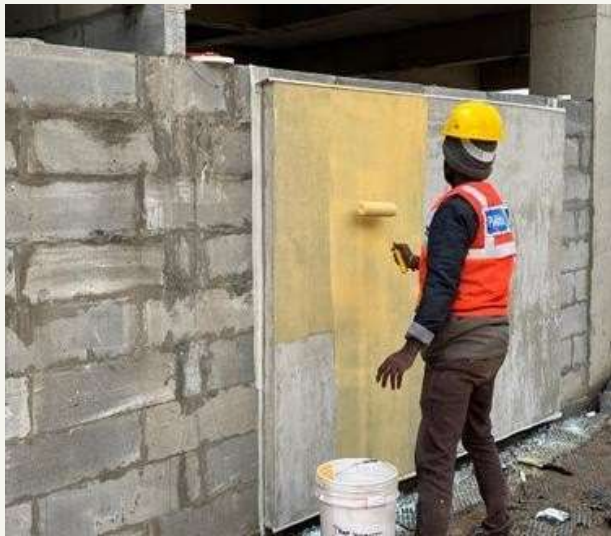
Applying primer for decorative finish
