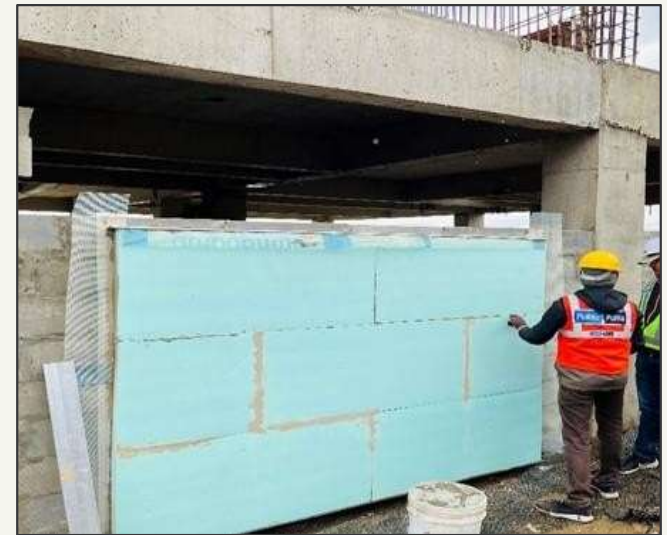
Fixing insulation panels
