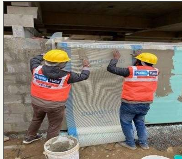
Applying Glass Fibre mesh
