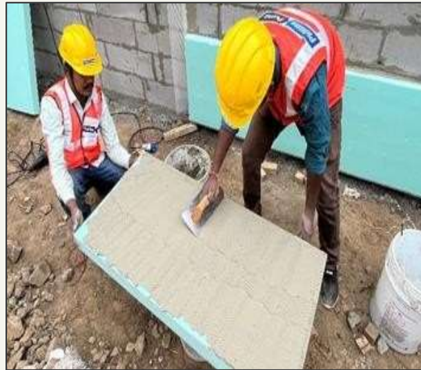
Applying Adhesive on the panel
