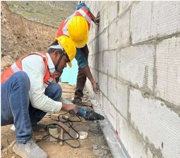
Fixing the starter profile
