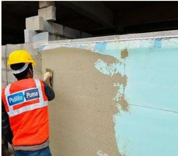
Applying First coat of mortar
