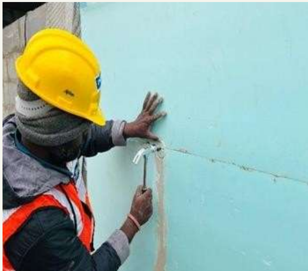
Mechanical Fixing with Anchors
