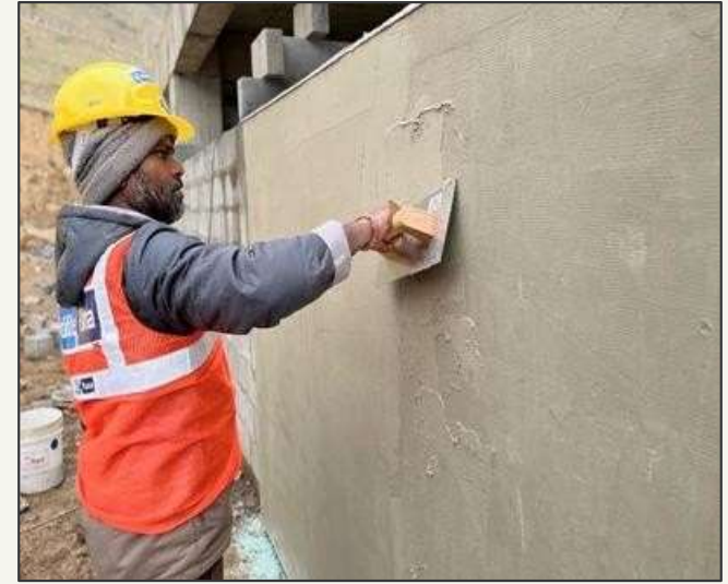
Applying second coat of mortar
