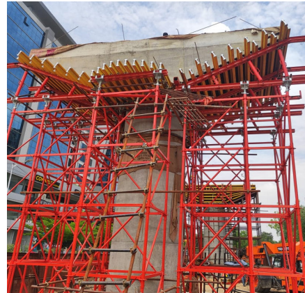
Pier Cap Support Bridge
