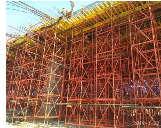
Metro and Highway Bridge Decks
