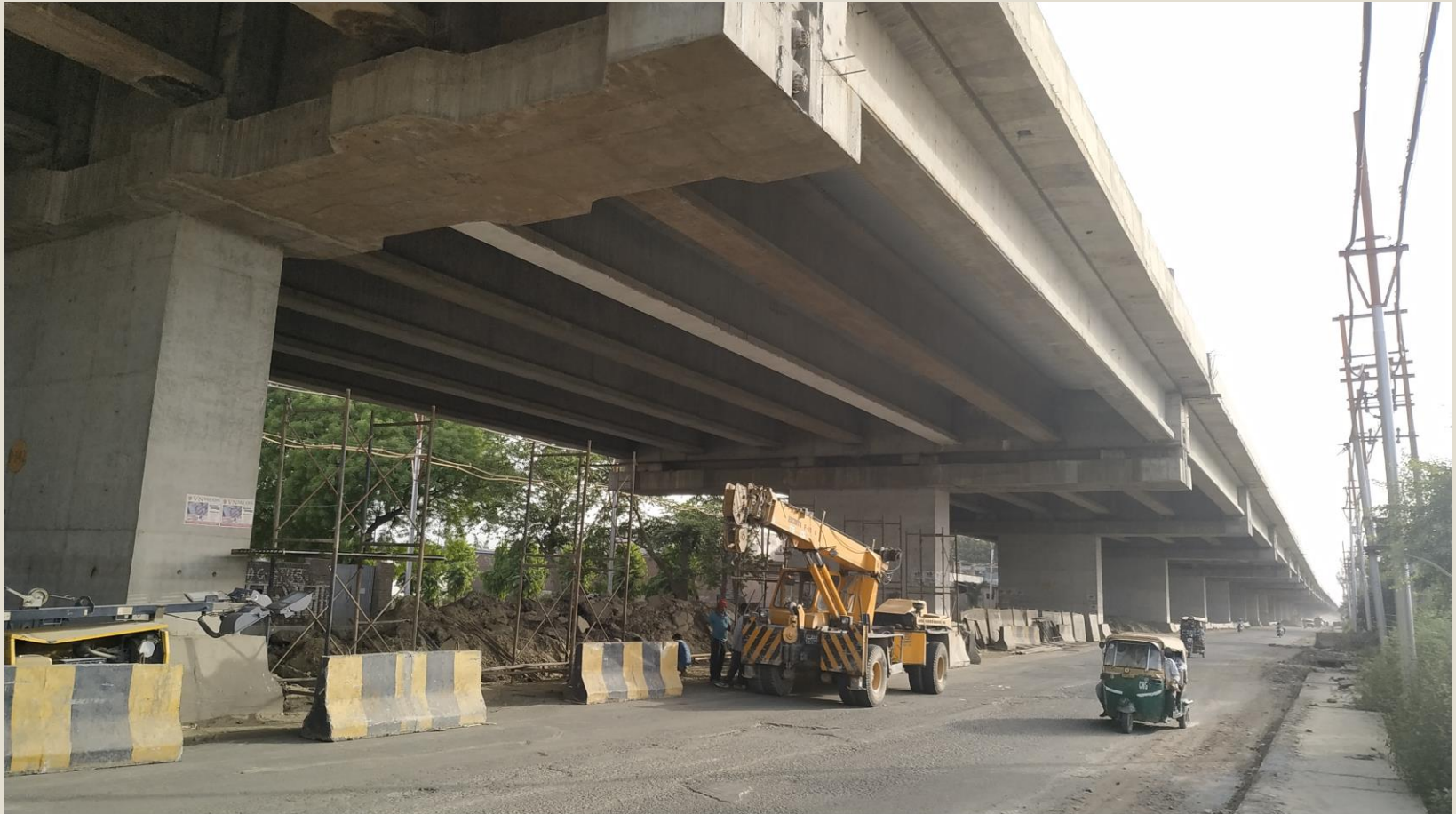
View of flyover
