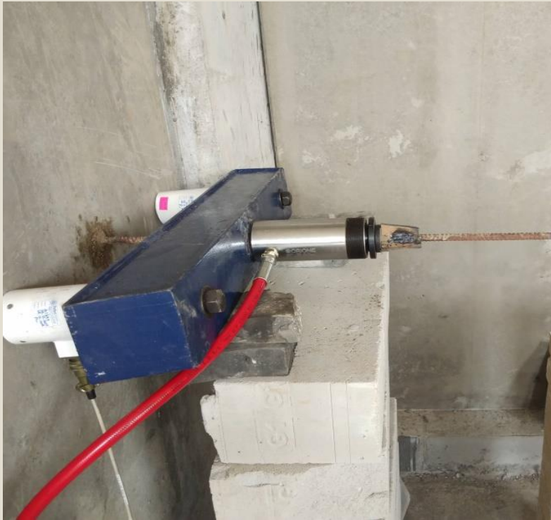
Pull-out test on Rebar Anchor
