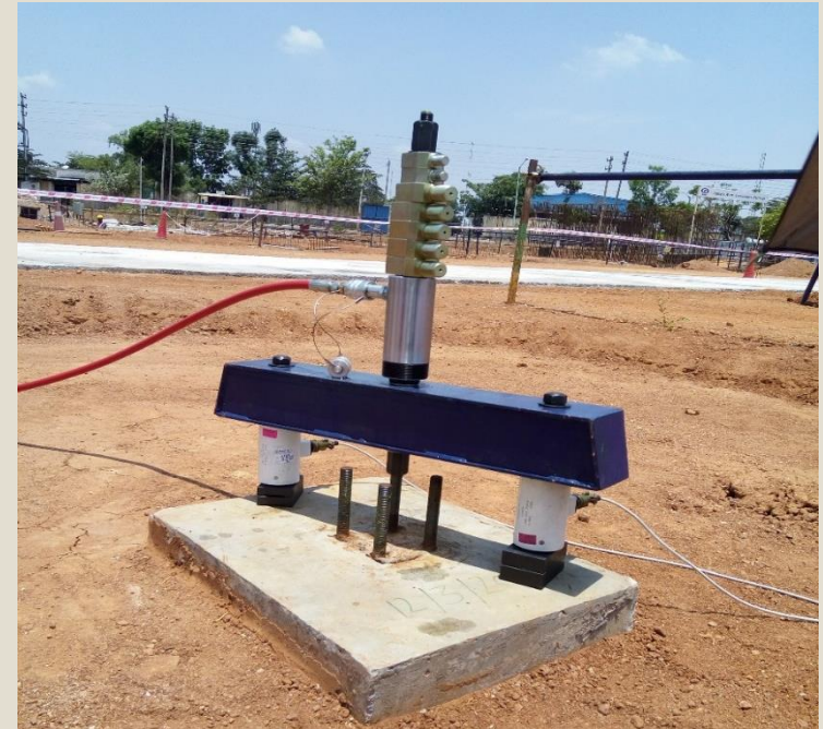
Pull-out test on Anchor bolt
