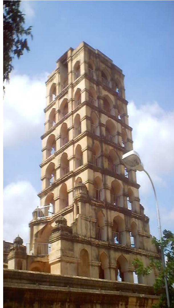
Multi-storeyed Un-reinforced masonry tower, Tanjavur, India
