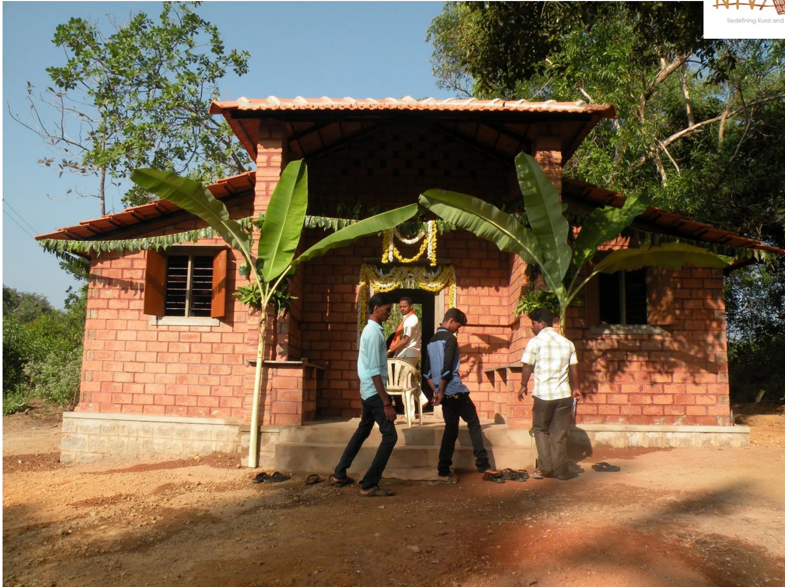
Interlocking blocks with thin-bed joint mortar, Cherkady, Udipi district
