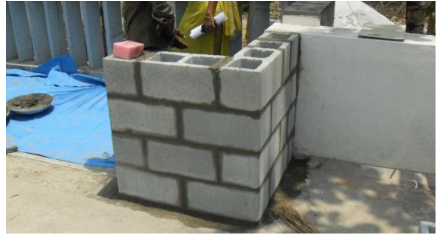
Retaining old Parapet wall and continuing construction with new technology.
