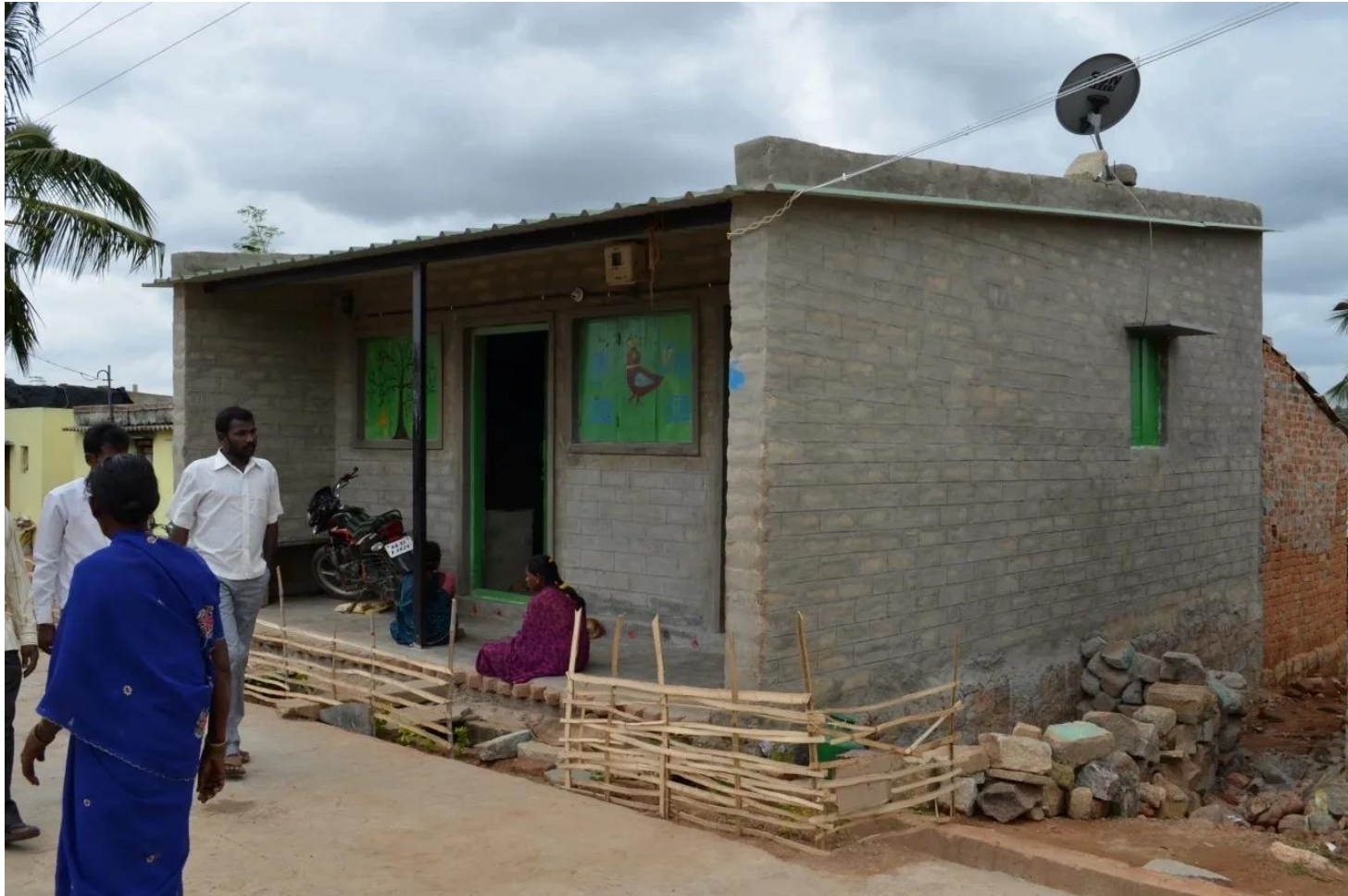
SAB technology at Thimmayannadoddi, Anekal taluk, Karnataka Technical inputs: Dr. Yogananda MR
