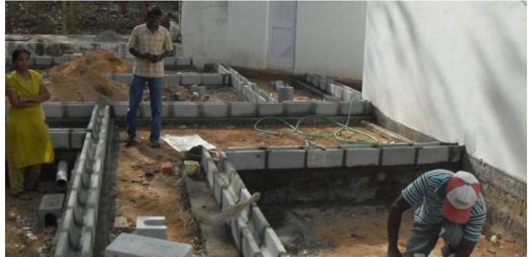
U-blocks laid to form beam structure
