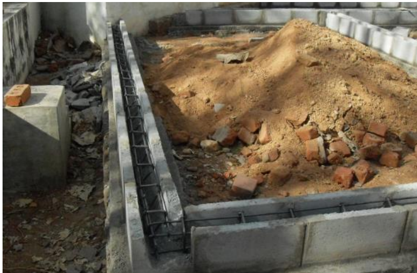
U-Blocks used for Plinth (and Lintel and Tie beams)
