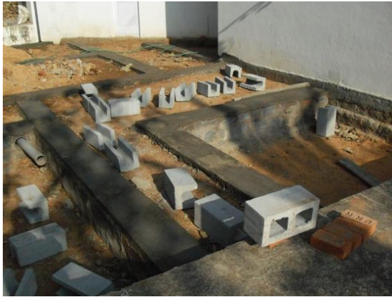
U-Blocks used for Plinth (and Lintel and Tie beams)
