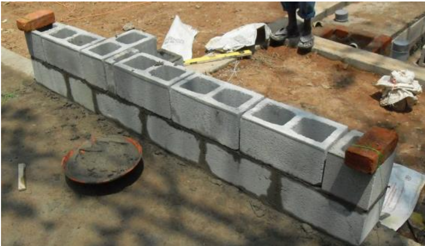
Lighter blocks help speed up construction!
