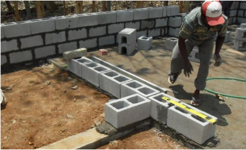
Wall construction on top of Plinth beam starts
