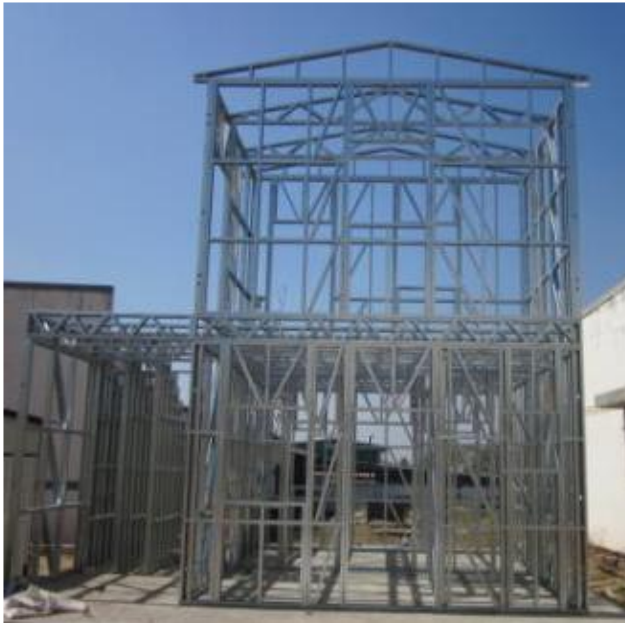
LGSEFS Infill Concrete Panel Demo Building at CTP for Full Scale Testing
