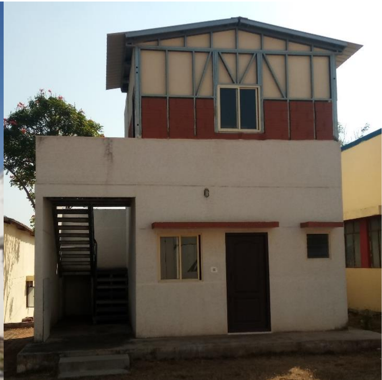
LGSEFS Infill Concrete Panel Demo Building at CTP for Full Scale Testing
