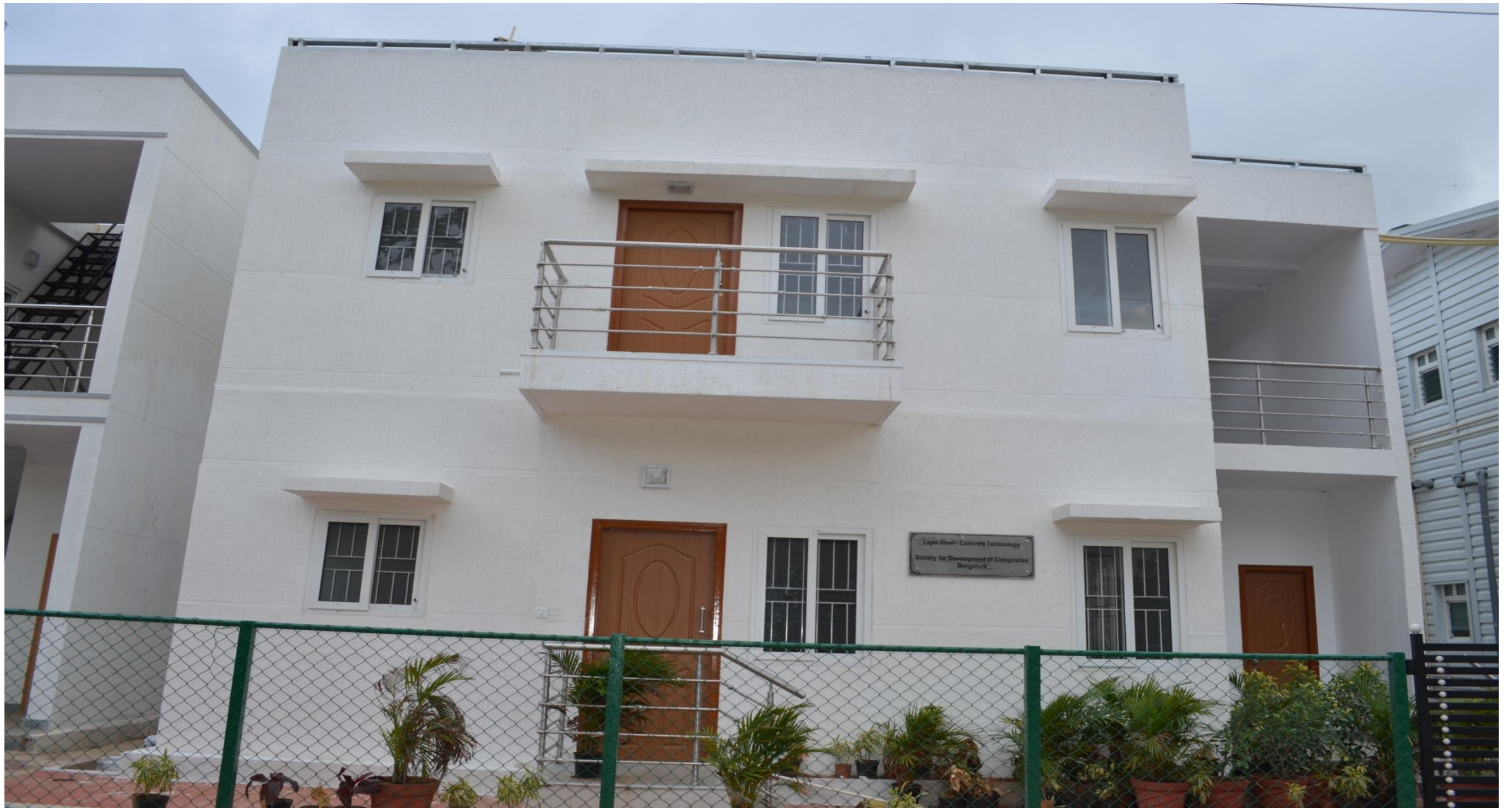
2 PC Quarters Constructed using LGSFS Infill Concrete Technology
