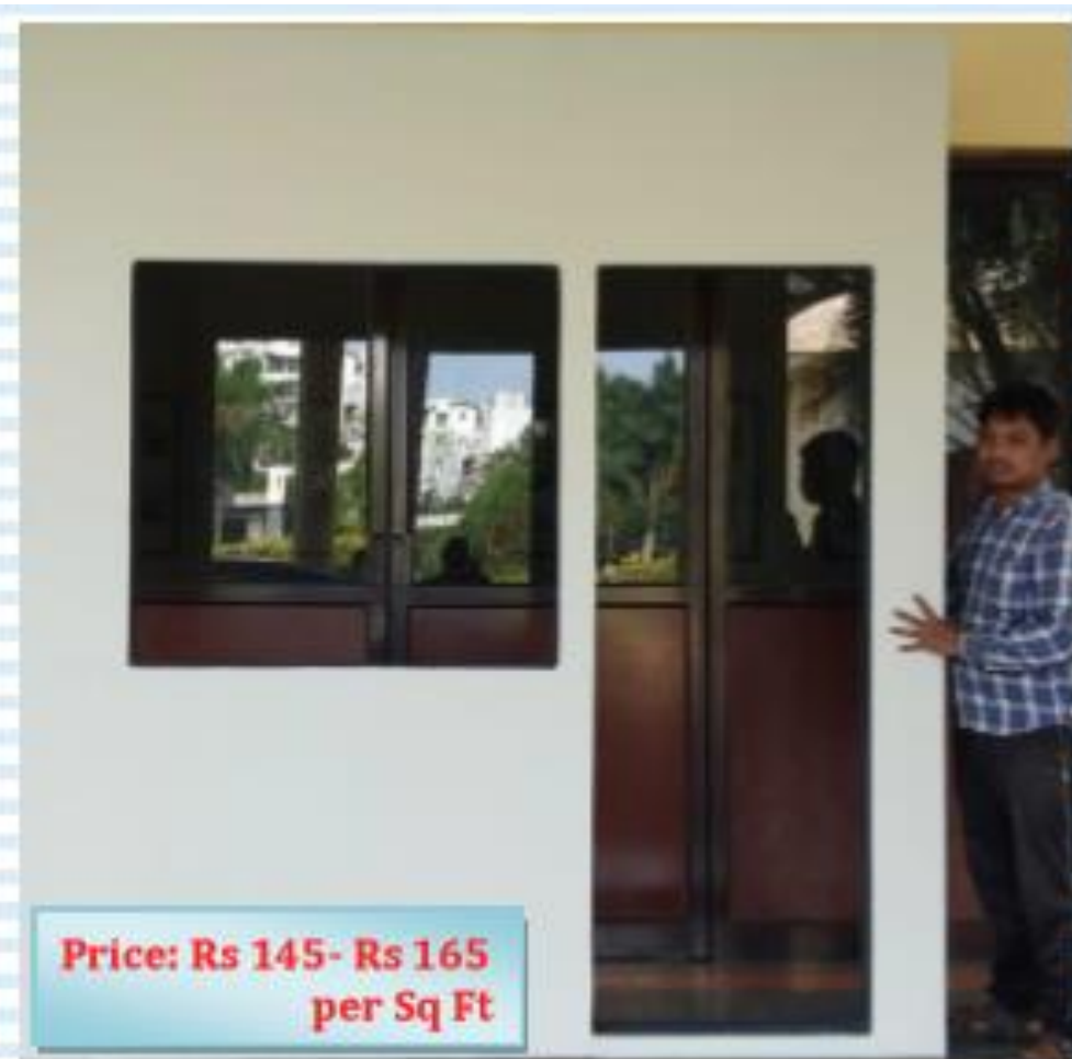
Steel Reinforced Sandwich Composite Load Bearing Wall with door & window openings Photo.
