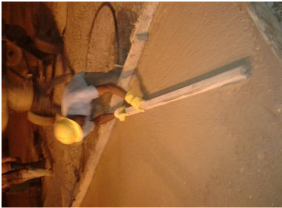
Surface levelling of GP Concreting
