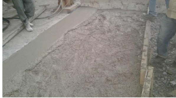
Img6 GP concrete casting at plotted area
