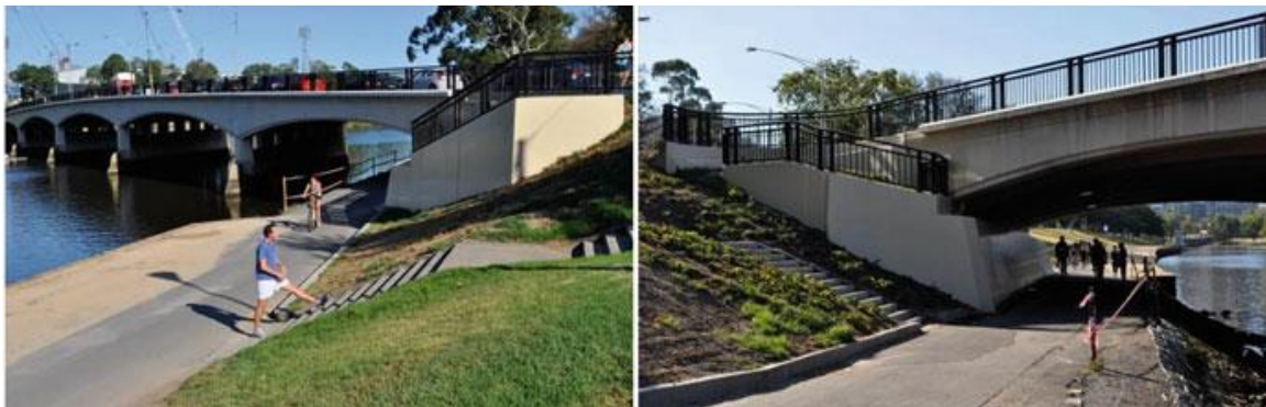
Fig. 5:E-Crete retaining wall at the Swan Street bridge in Melbourne, Australia
