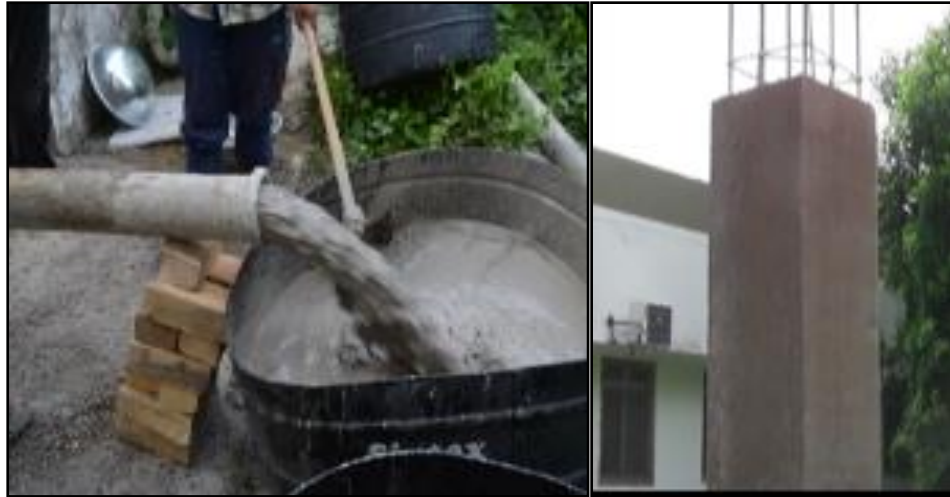
Fig. 7. Self-compacting geopolymer concrete and its casted column
