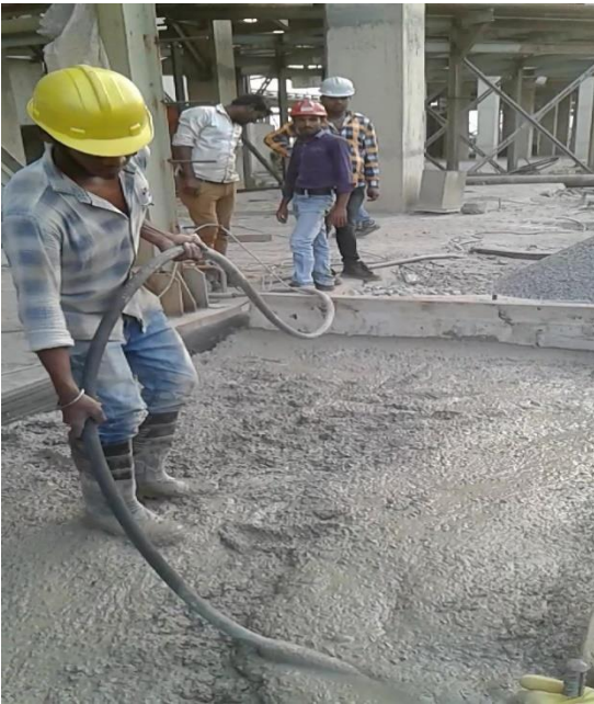
Img5 220mm slump without segregation
