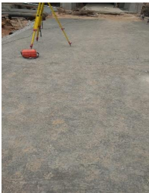
Surface levelling of GP Concreting
