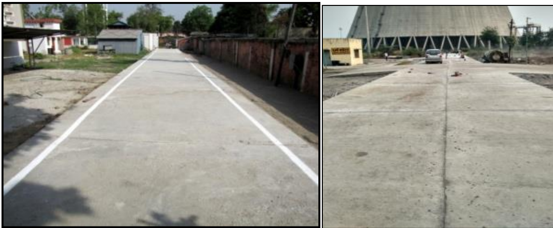
Fig. 8. Geopolymer concrete roads(a) 50 m at CSIR-CBRI, Roorkee (b) 100 m at NTPC Dadri
