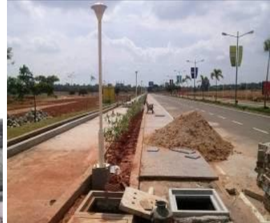
Pavements / Roads at Ozone Urbana Bangalore
