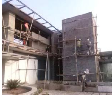
Roads & Canteen Building at ACC Kuttini
