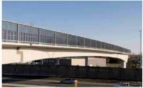
Glenmore/Legsby pedestrian bridge, Calgary, Alberta, Canada
