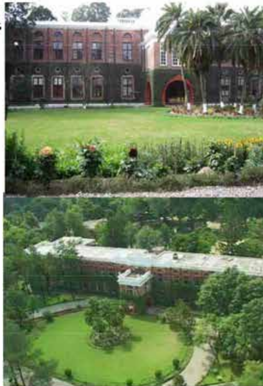
Doon school drastically reduced the need for artificial heating/cooling air conditioning through solar thermal systems and cross-ventilation
