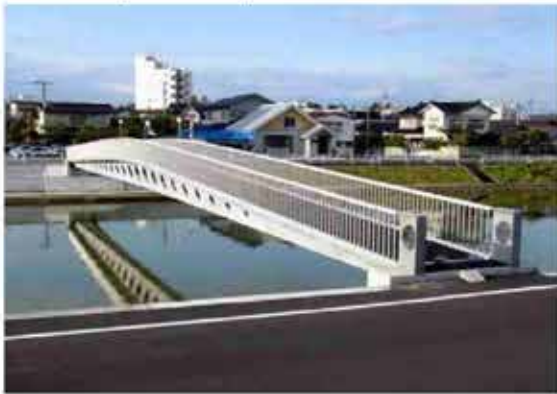
Sakata-Mirai bridge, Sakata, Japan
