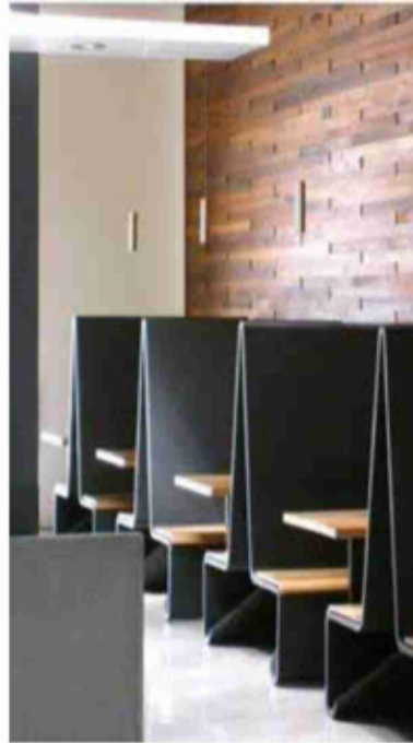
Super thin structural concrete - Ductal - is used in the Bar Agricole in San Francisco
