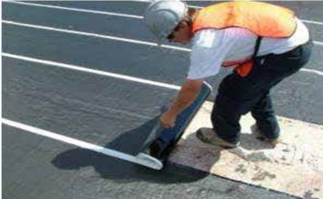
Polyisobutylene (PIB) :Glazing Sealants,Waterproof Membranes
