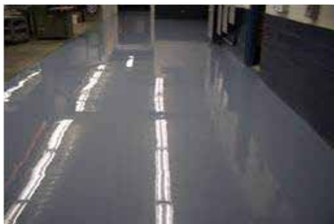
FLOOR AND HANGER COATINGS,
