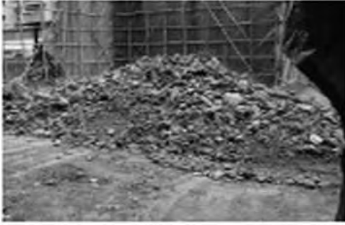
8. Sorted broken concrete stockpiled separately
