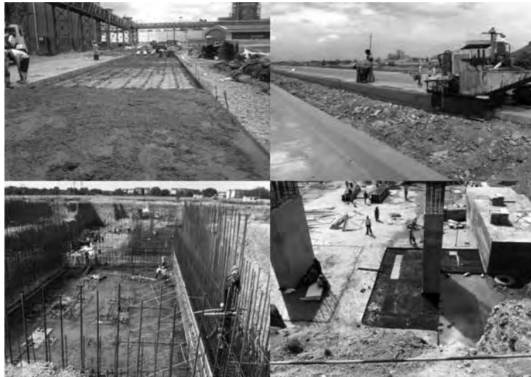
Fig 4: Usage of granulated BF slag and crusher dust at JSW Vijayanagar works
