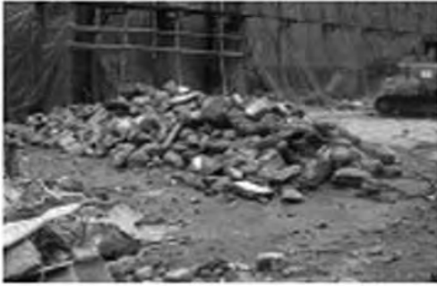
9. Sorted broken concrete stockpiled separately.
