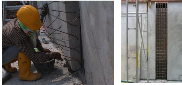
Figure 11 — Preparation for Grouting and Vertical Connection Post Installation of Precast Components
