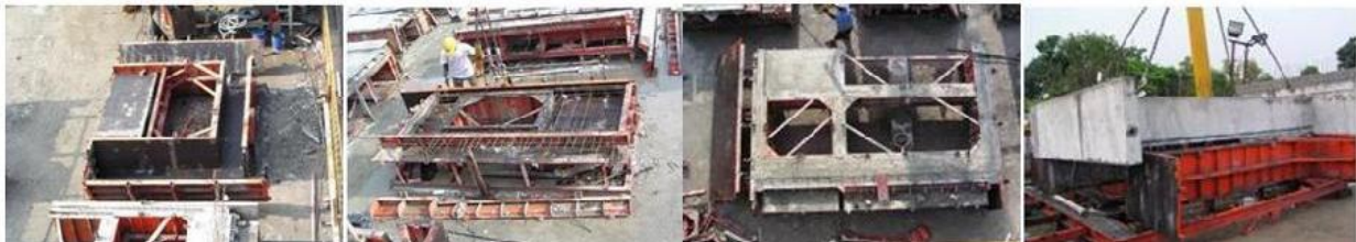
Figure 4 — Various Operations In The Production Yard During Production of Façade Elements
