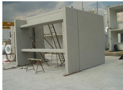
Figure 2 — Precast Bay Window and Walls
