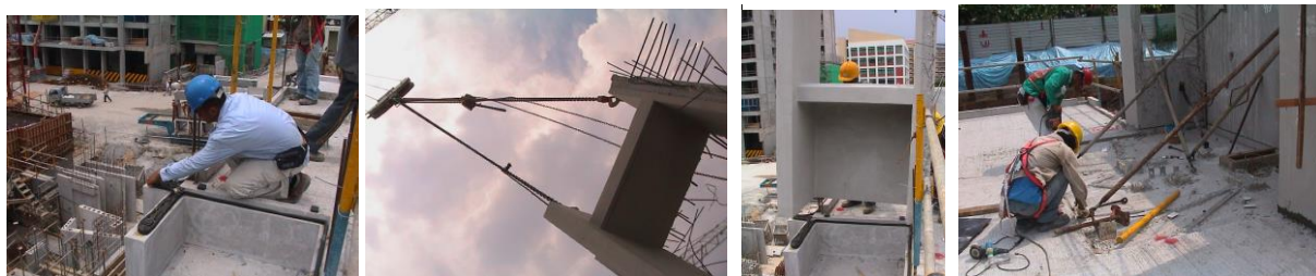
Figure 10 — Various Operations During Installation of Precast Components
