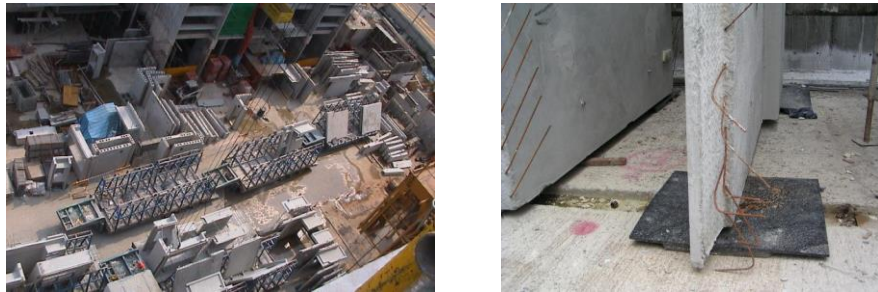
Figure 9 — Delivery and Storage of Precast Components at Site
