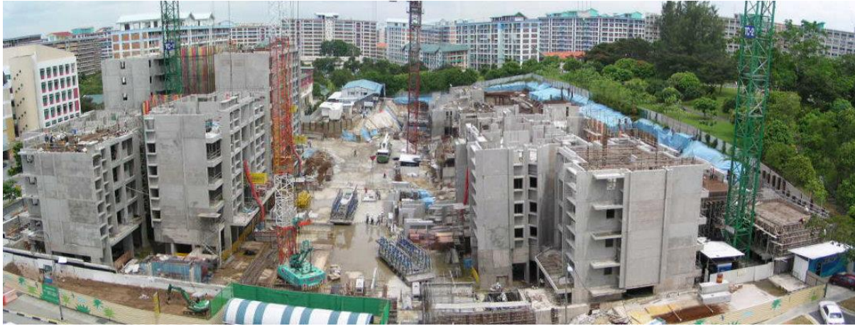
Figure 3 — The Esparis Executive Condominium Under Construction
