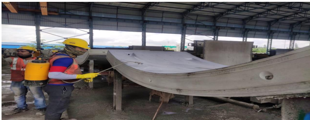
Application of curing compound after demoulding
