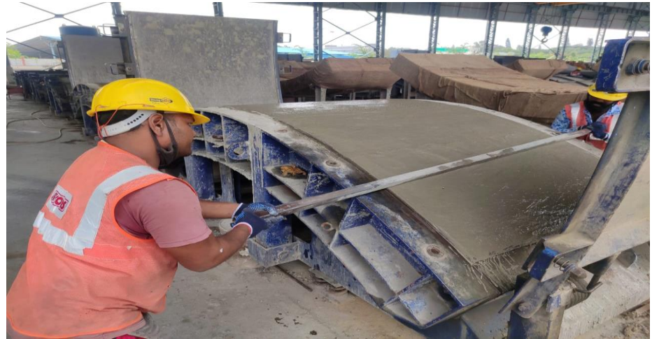
Finishing of extrados face
