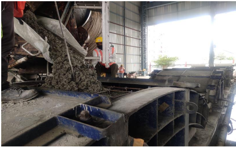
Concreting after placing cage on mould
