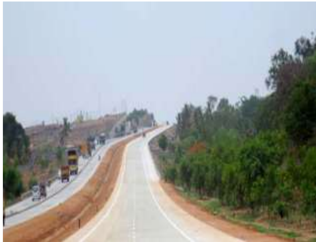
Rigid Pavement Construction (Composite Type), Bangalore- Mysore Infrastructure Corridor Project (BMICP)
