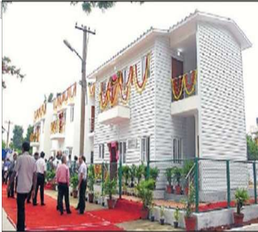
Construction of 2 PC Quarters for Karnataka State Police Housing Corporation Limited (KSPHCL), at Adugodi, Bangalore.
