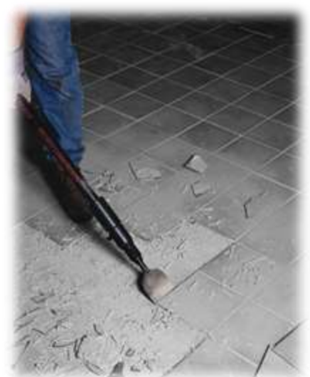
Flooring and tiling
