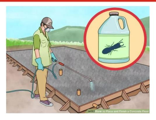
Pretreat the fill and subgrade for insects using an approved and labeled termiticide. This is usually done by a bonded and licensed pest control company
