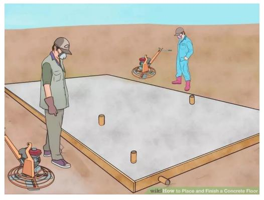
Let the concrete continue to set after it has been troweled the first time. If the surface is flat and free of defects, you can allow the concrete to harden until it is ready for the finish troweling. Because the concrete is placed in a continuous operation, the first area that is poured will normally set up first, but be aware that areas exposed to hot sun or wind may get hard earlier than areas that were placed in a shaded, protected location.
