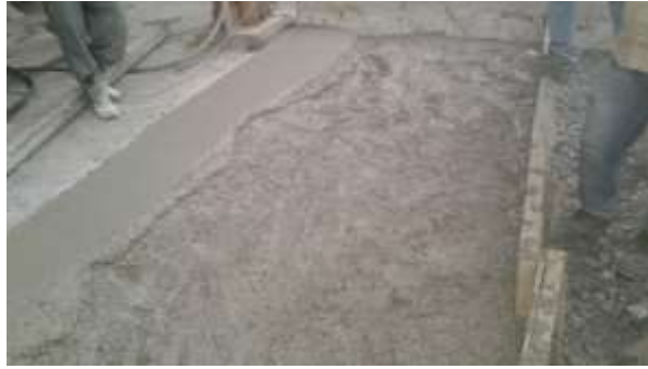
Img6 GP concrete casting at plotted area
