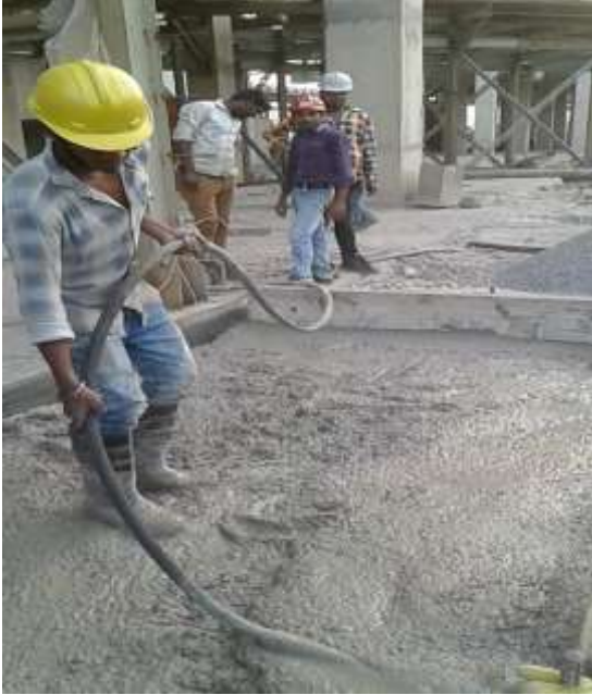
Img5 220mm slump without segregation
