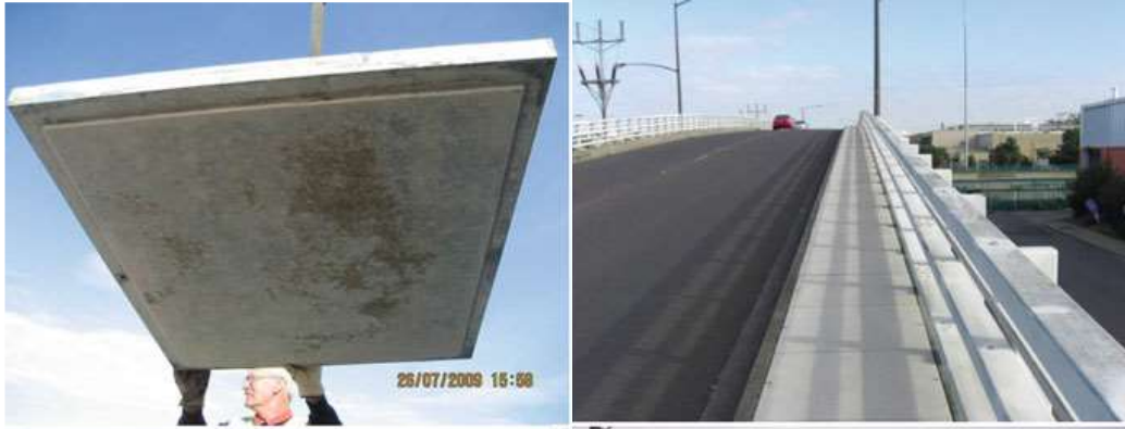
Fig. 4:E-Crete pre-cast footpath at Salmon Street bridge in PortMelbourne, Australia
