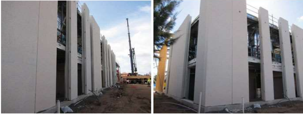
Fig. 2: Precast geopolymer concrete panels for Melton Library, Melbourne, Australia
