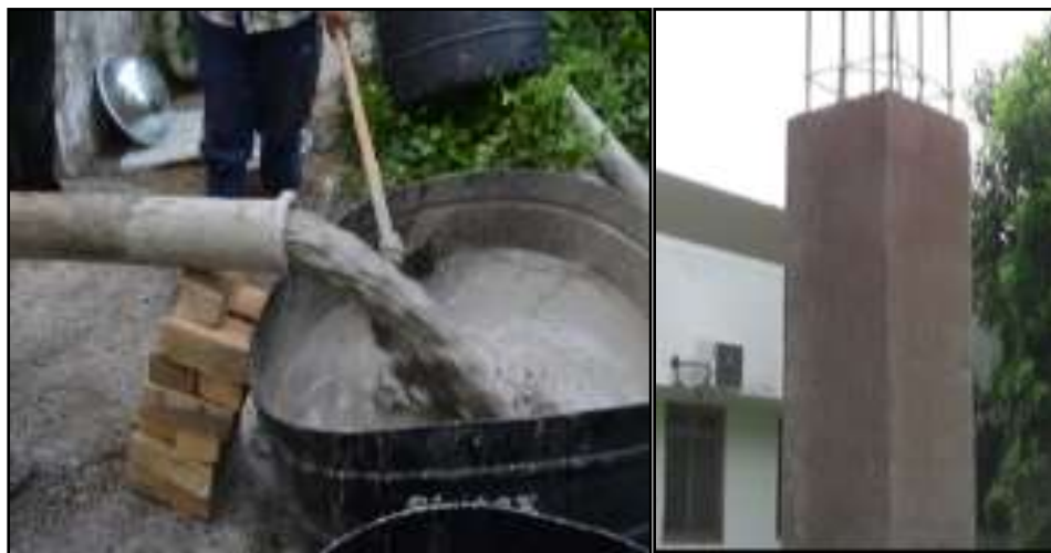
Fig. 7. Self-compacting geopolymer concrete and its casted column
