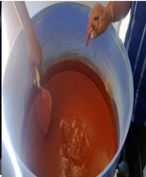
Wet mixing of geopolymer composite
