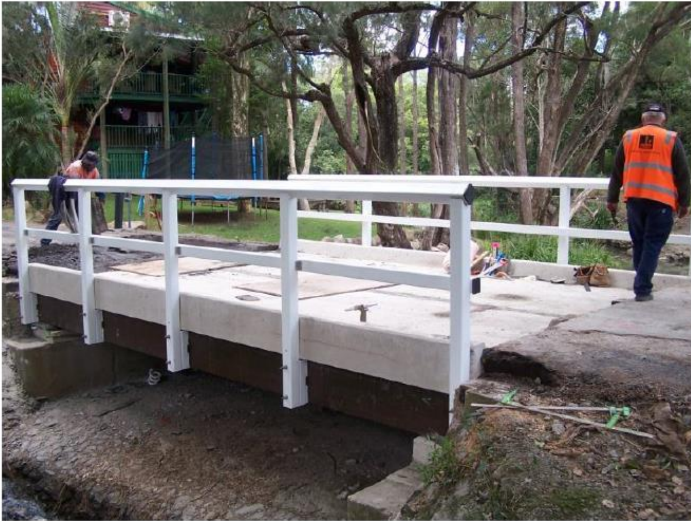
Composite pultruded girder and Grade 40 geopolymer deck bridge in Brisbane.
