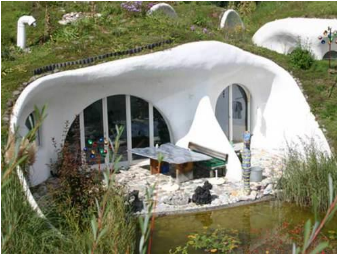
STONE ARCHES WITH GEOPOLYMER FERRO CEMENT
