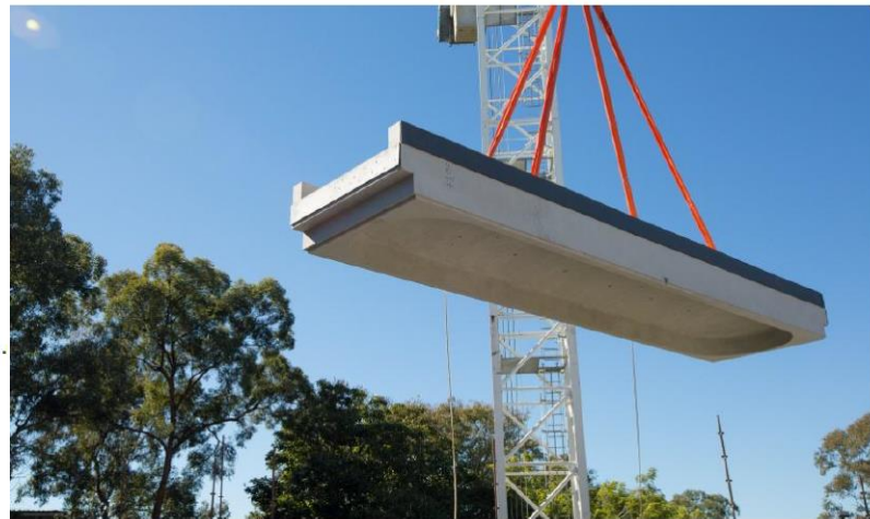
10.8 metre geopolymer beam with vaulted soffit being craned into position.
