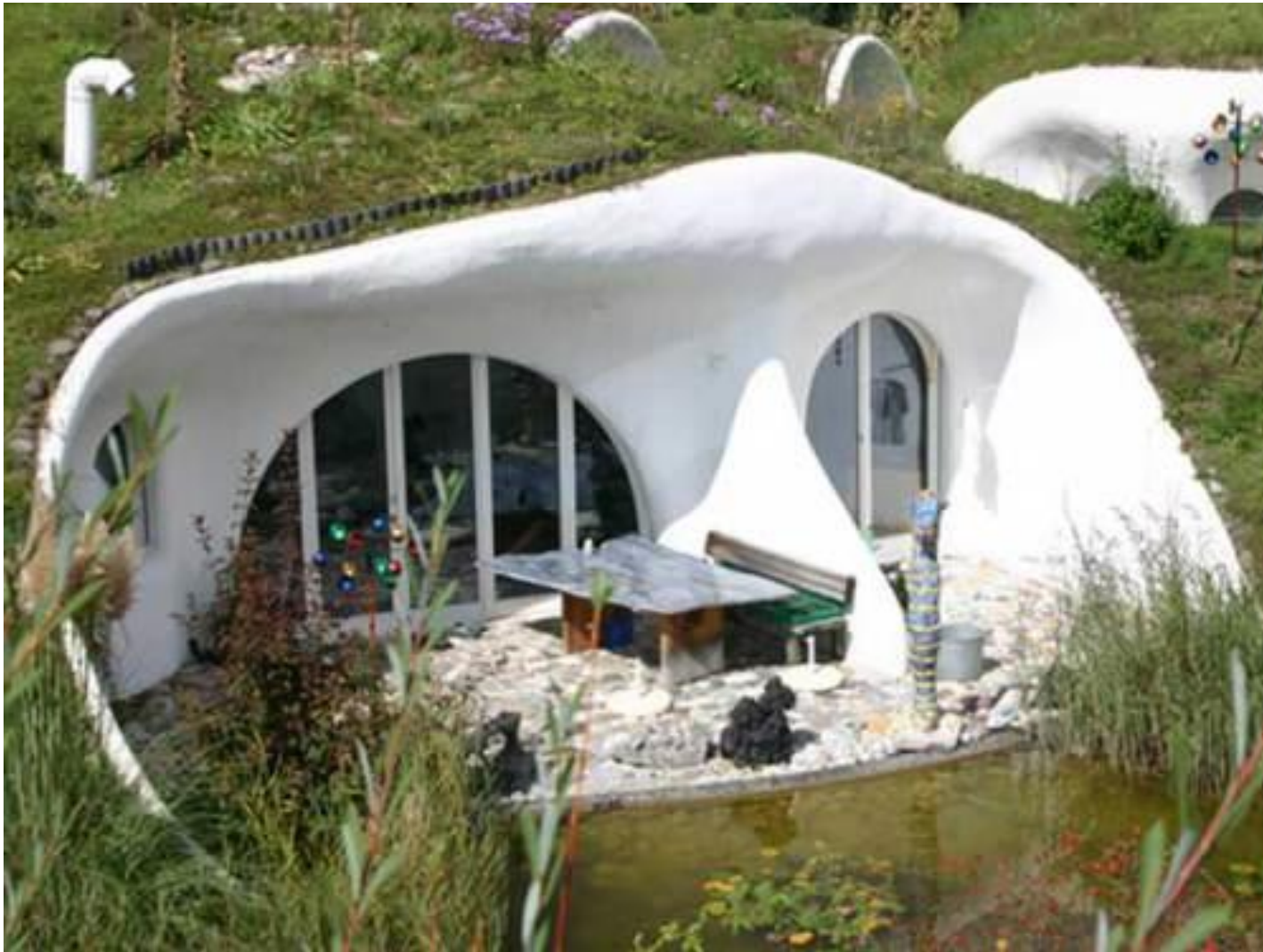
STONE ARCHES WITH GEOPOLYMER FERRO CEMENT
