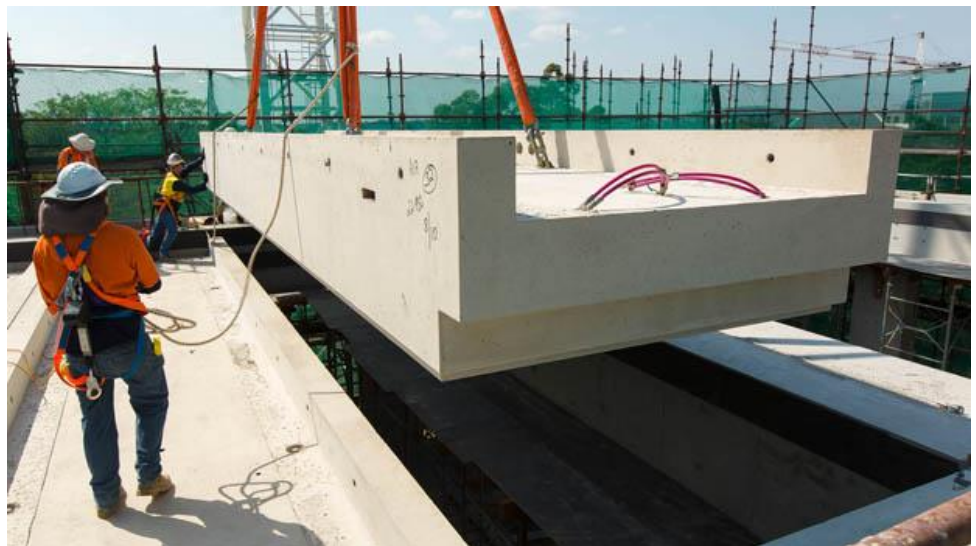
10.8 metre geopolymer beam with vaulted soffit being craned into position.
