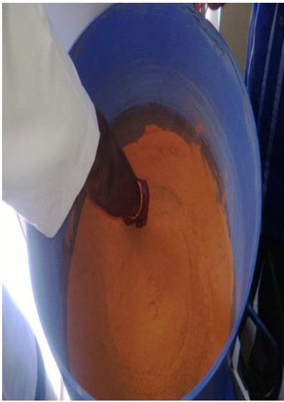
Dry mixing of materials
