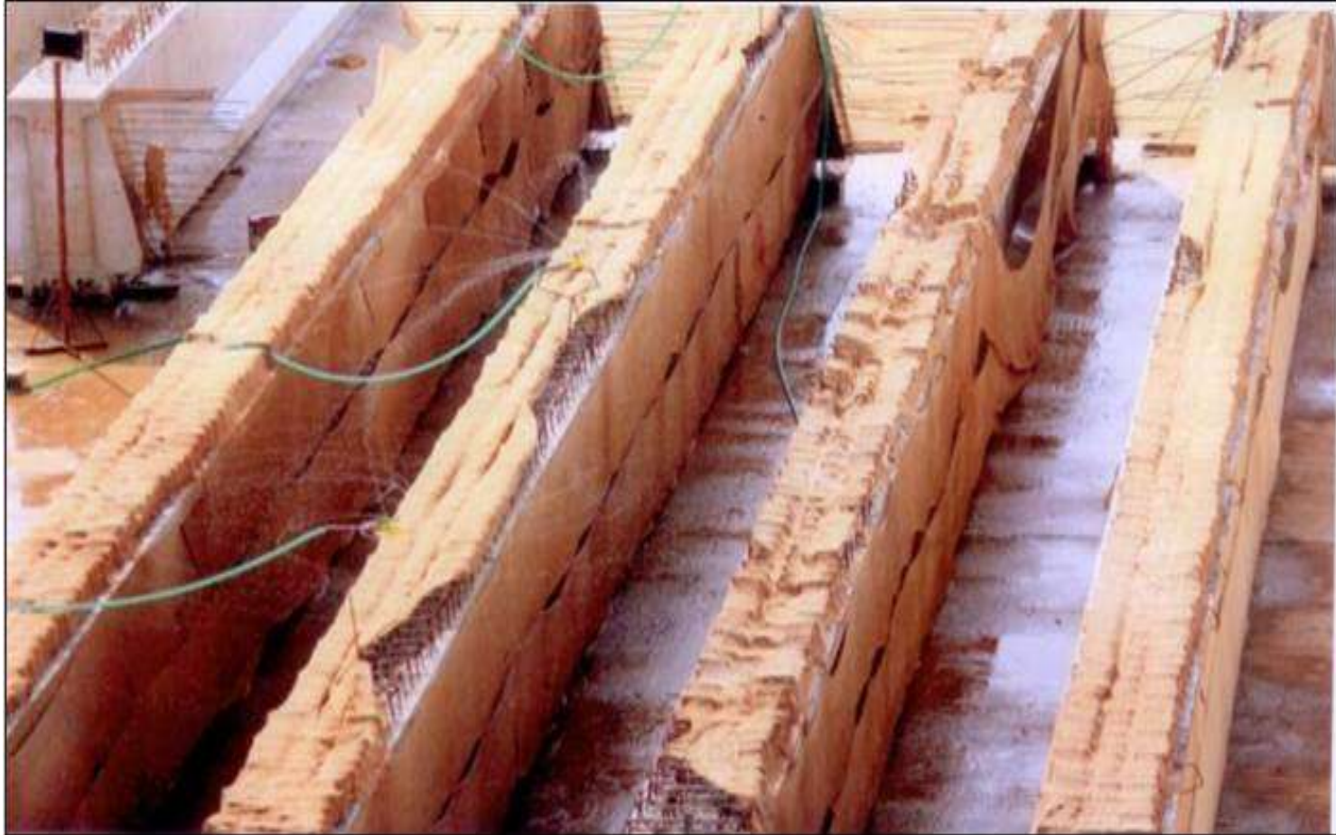
Fig.16 : Curing of precast I Girders, 24 x 7 with Water by Sprinklers.
