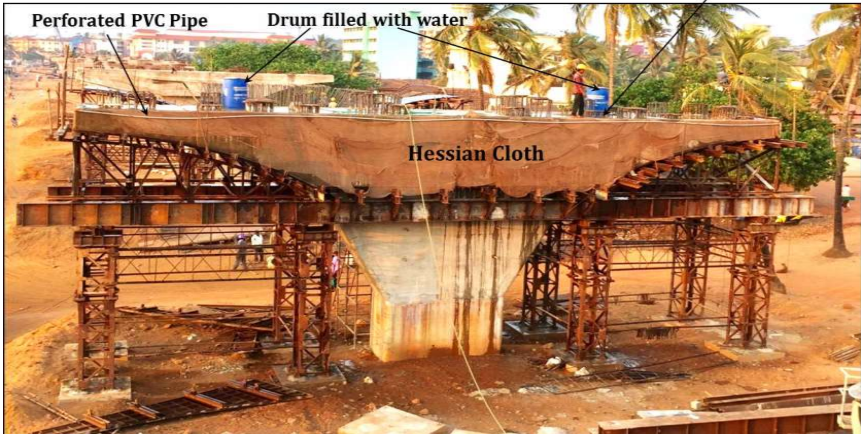
Fig. 13 : Curing of Pier Cap, 24 x 7 by Water
