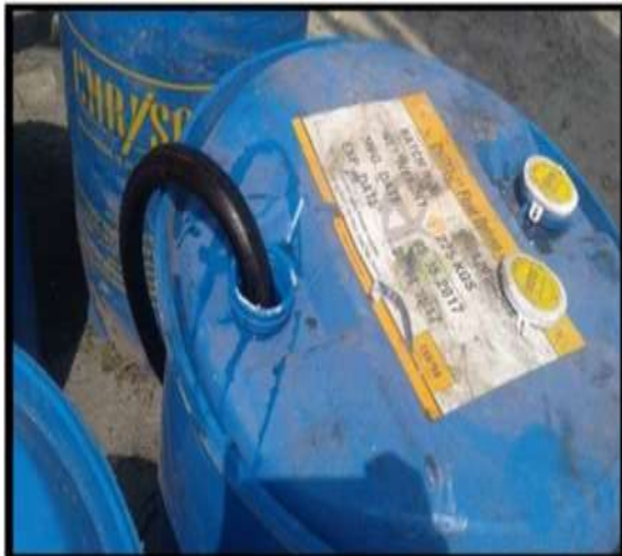
Incorrect Method – Cap to be provided to arrest dust contaminating the chemical
