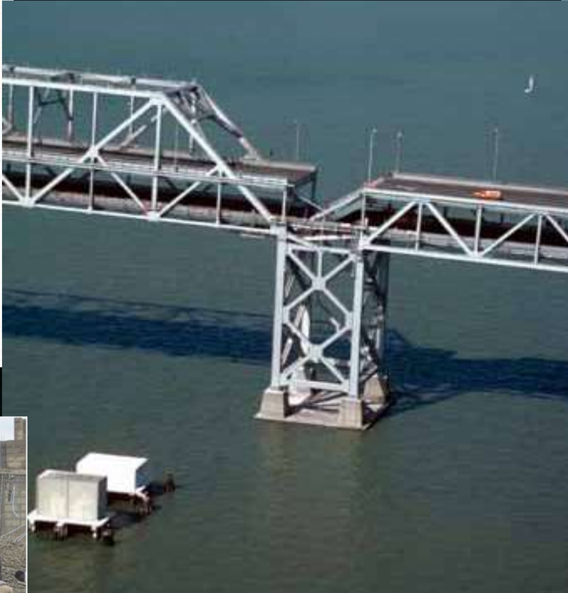
Structural Element Failure
