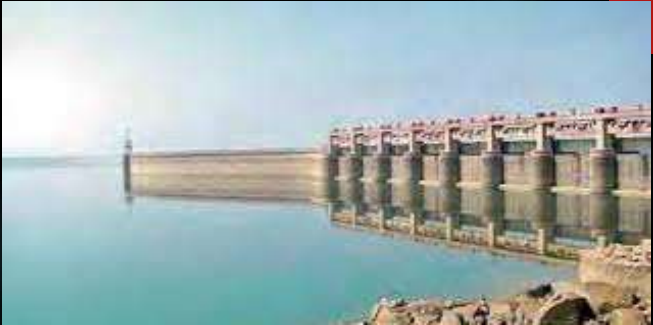
KRS Dam, Karnataka
