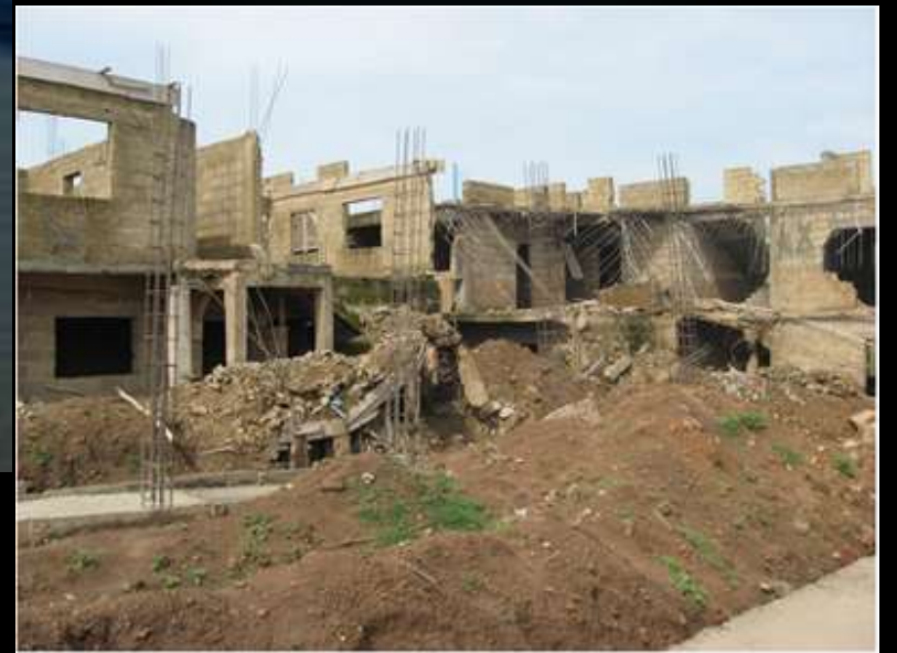
Wall-structure Failure
