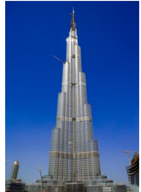
The Burj Khalifa (United Arab Emirates) is the tallest man-made structure ever built. It is supported by a reinforced concrete core using a special concrete mix.
