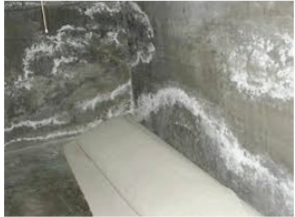
Salt Efflorescence
