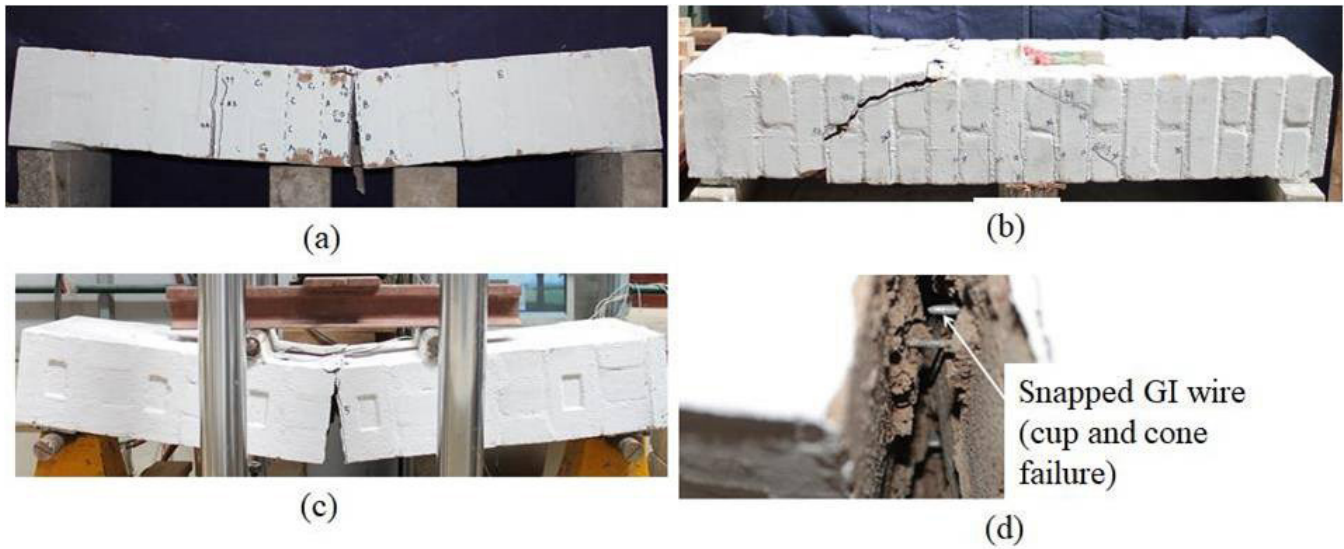
Figure 8. Failure pattern of the (a) EB1 (b) EB3 (c) Rtb and (d) snapping of steel
