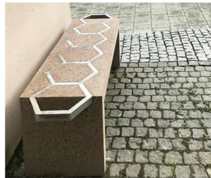
Aluminium Reinforced bench
