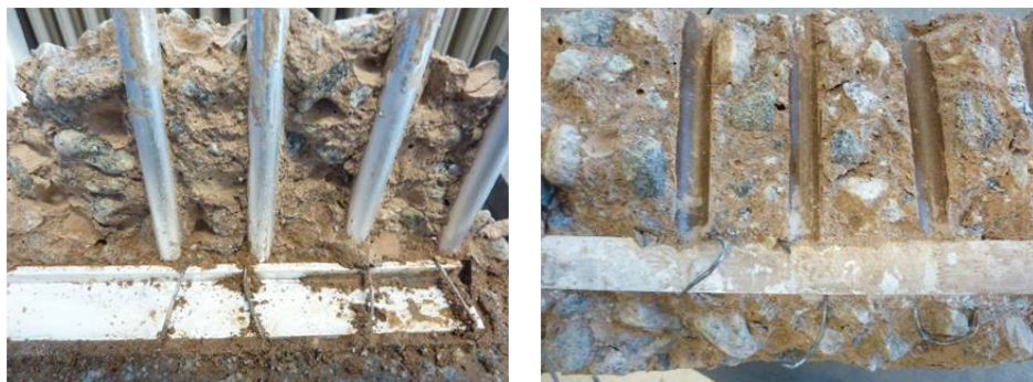
Fig. 5 - Split concrete beam at 40 days age showing that aluminium bars (left image) are not corroded (including a T-profile bar in same alloy perpendicular to them) and that the imprints in the concrete (right image) are free from corrosion products.
