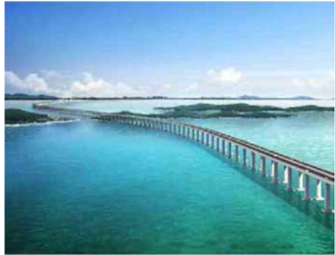
Figure 8 Temburong Bridge project
