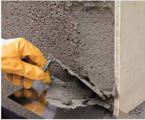
Figure 6: Filling of affected / honeycombed areas
