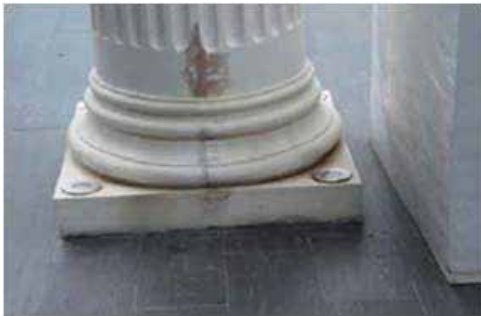
Fig 9. View of 13th Floor deck slab floor near pillar
