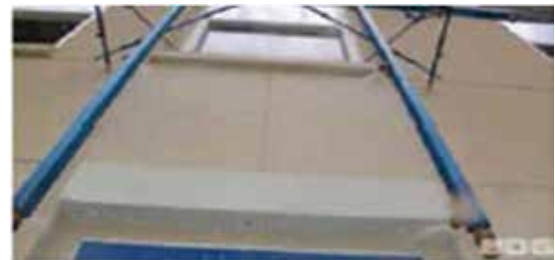
Fig.2 Leakage test by pipe spray system at external wall
