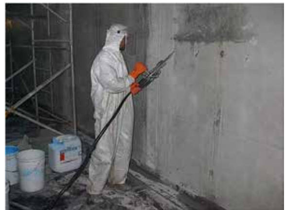
Figure 5: Addressing Leaking Cracks by Injections
