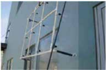
Fig. 1: A field leakage test by pipe rack system at window frame
