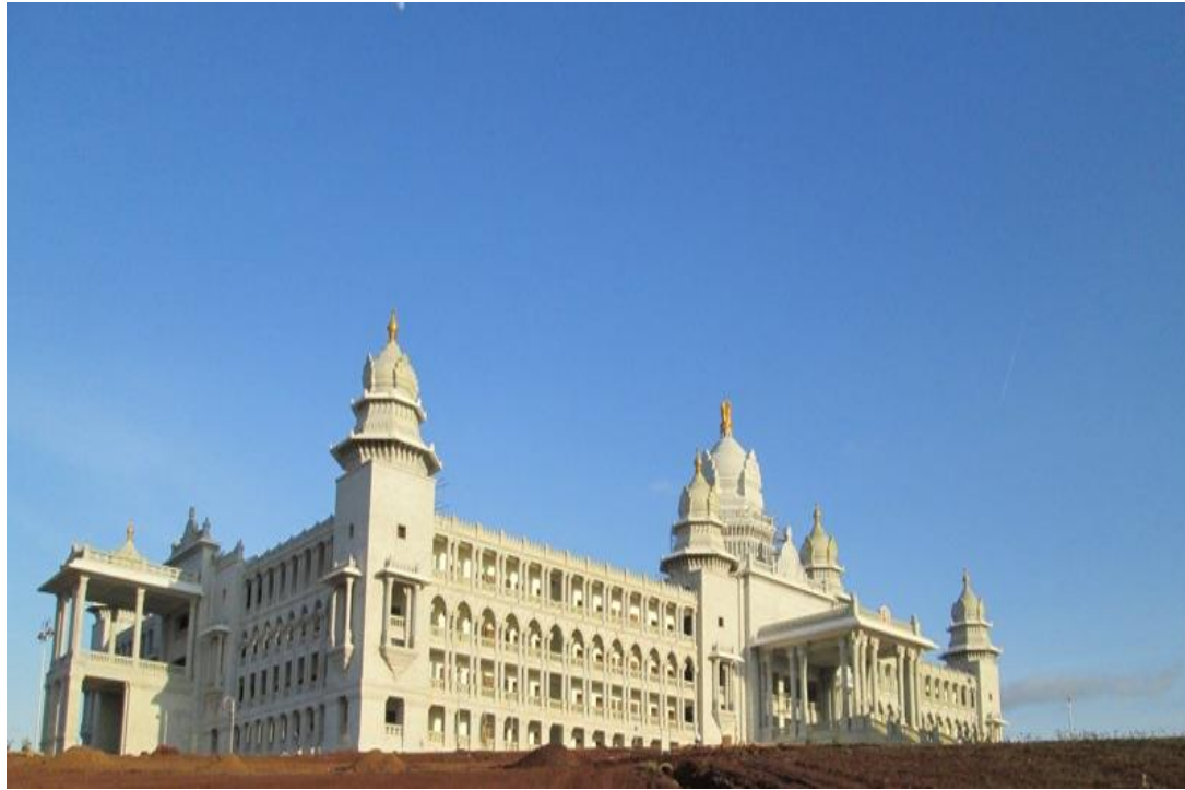
*Suvarna Soudha building , Belgaum,Karnataka,was awarded the ICI-KBC-Birlasuper Endowment Award for outstanding Concrete Structure of Karnataka 2012.
